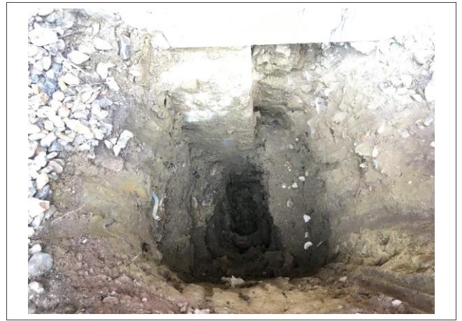
20: HDP4 right of drain
