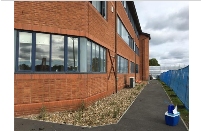
01: East wall of Building 124 facing north
