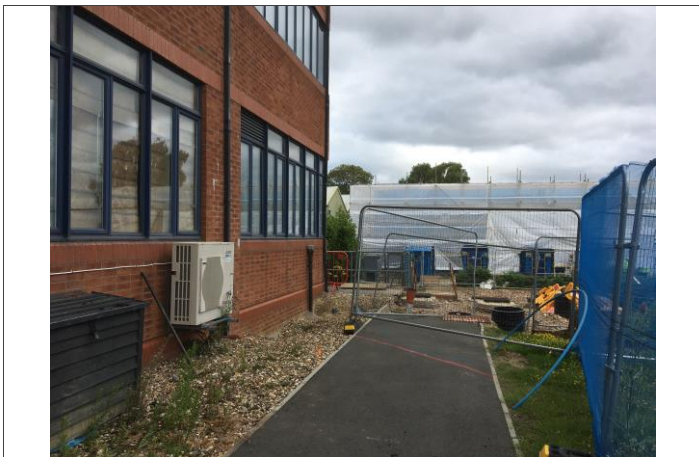
03: Northern part of Building 124 facing north
