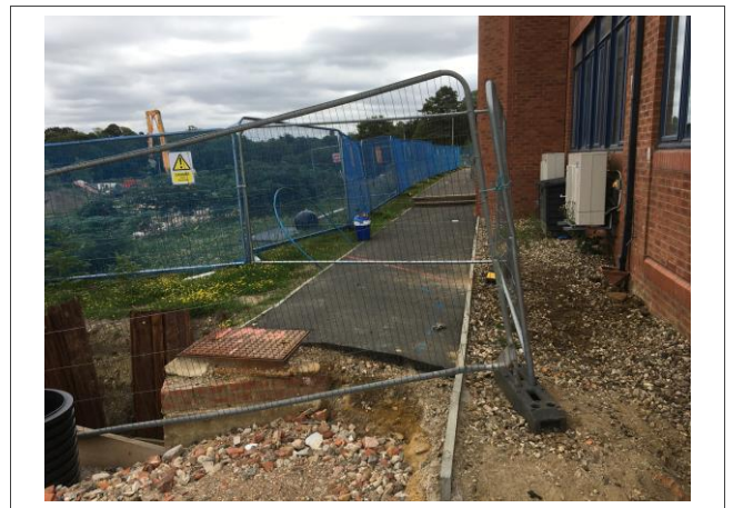
04: Northern part of Building 124 facing south
