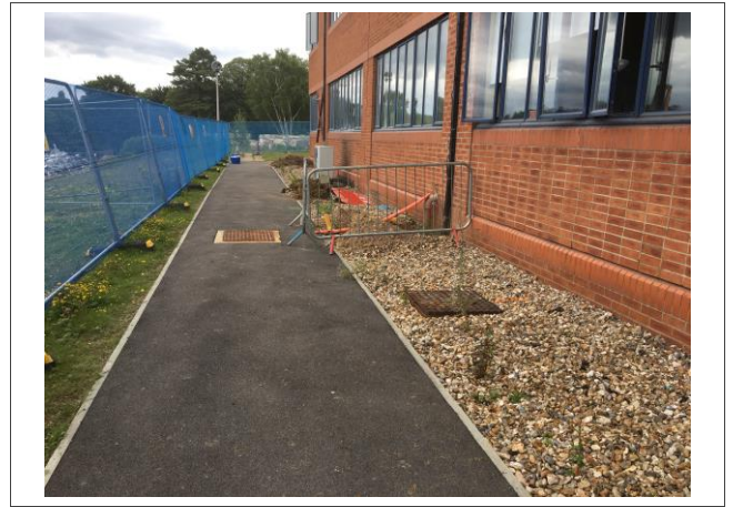
02: East wall of Building 124 facing south
