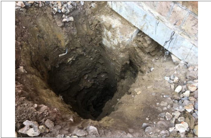
19: HDP4 right of drain
