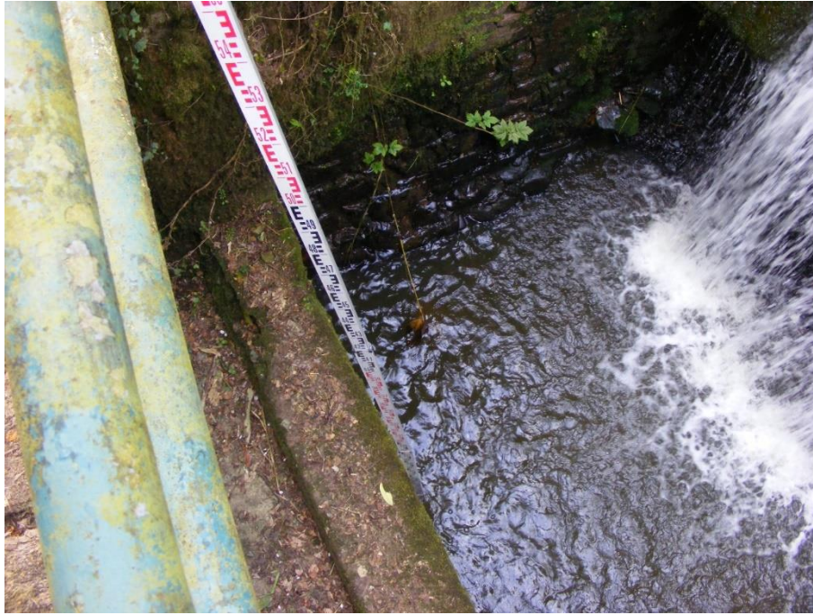
Figure 5: looking down into the weir pool from the footbridge.
