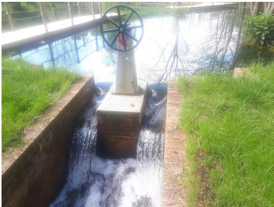
Figure 1: mill pond spillway weir.
