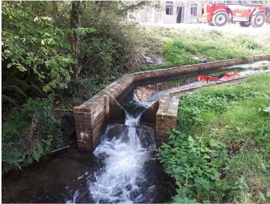
Figure 2: v-notch set up on tailrace weir (Levelogger attached to upstream wall).
