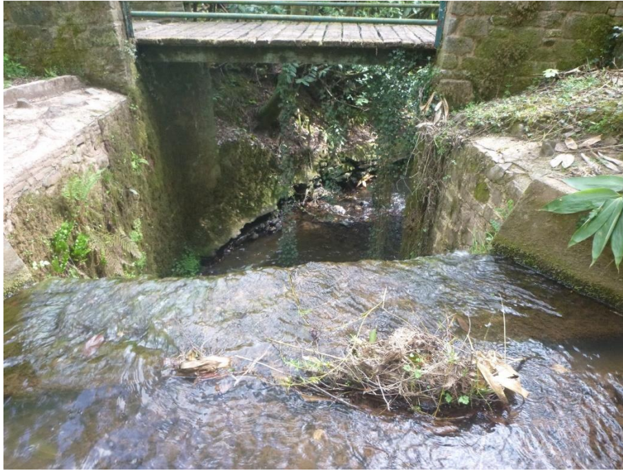
Figure 3: weir viewed from the upstream end.
