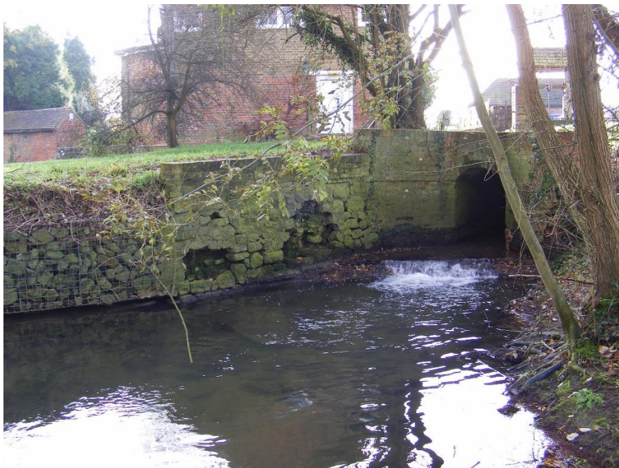
Figure 4: Outfall from bypass sluice channel.
