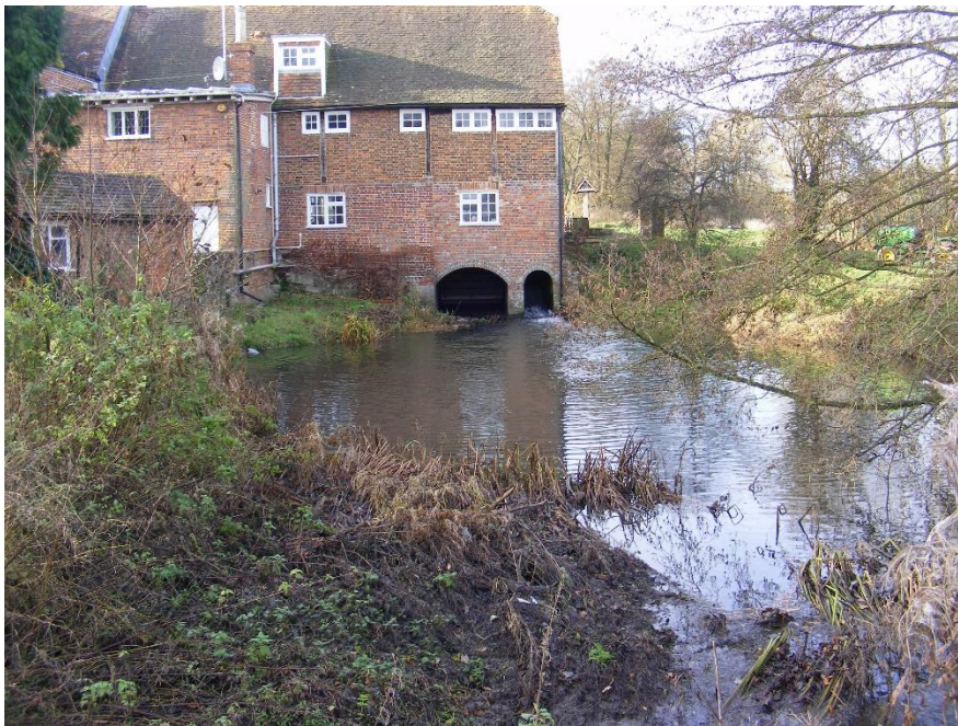
Figure 1: view looking upstream toward the mill, proposed turbine location to the right of the building.
