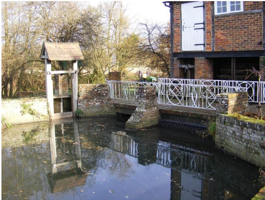
Figure 3: Looking downstream toward bypass sluice on the left (proposed intake location) and redundant mill wheel channel to the right.
