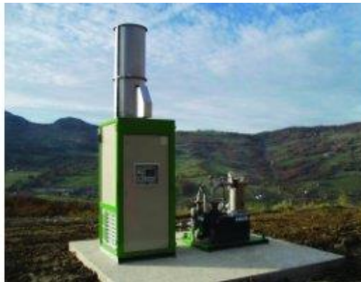
Figure 11.9: Example Enclosed Incinerator
