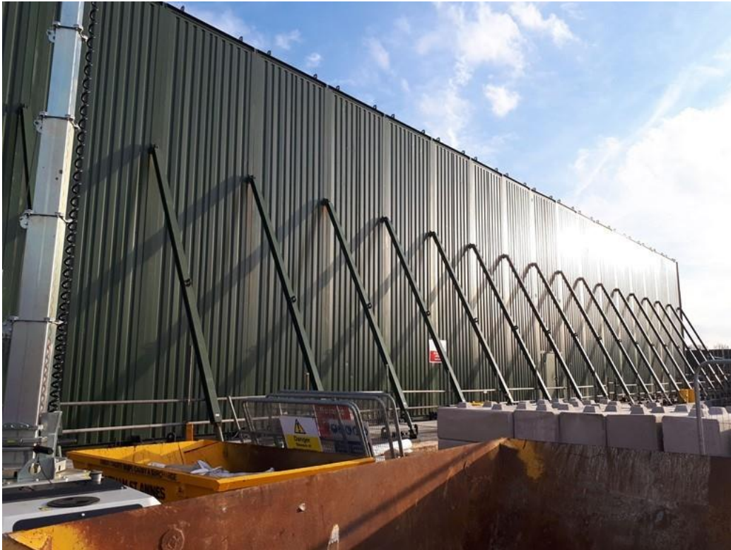
Figure 11.6: Example Demountable Acoustic Barrier
