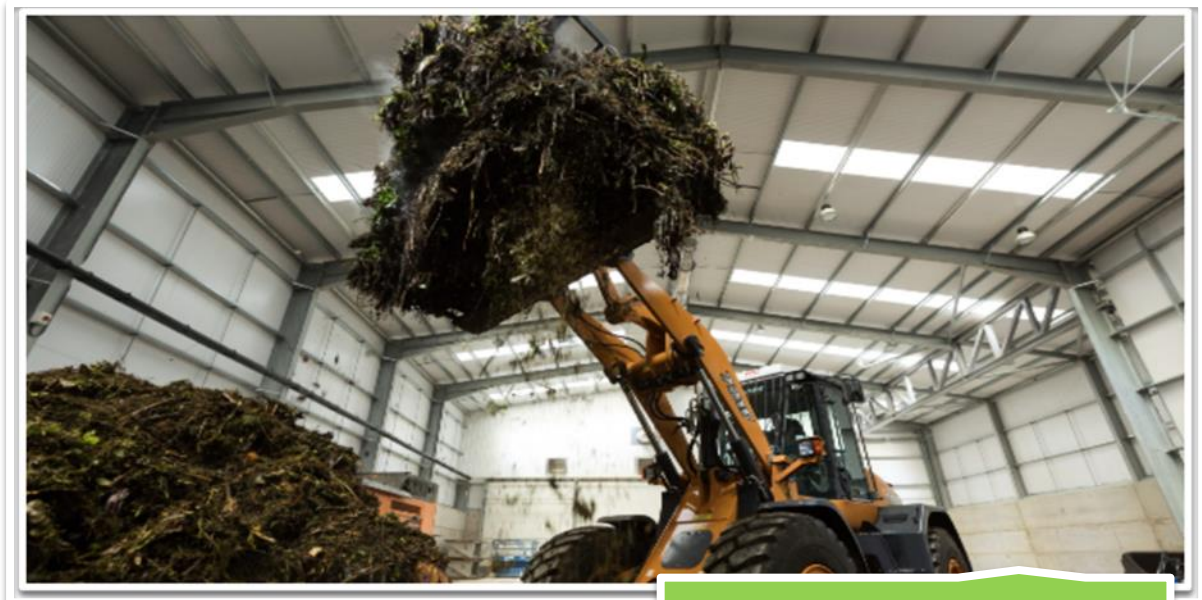
Willerby IVC Facility
