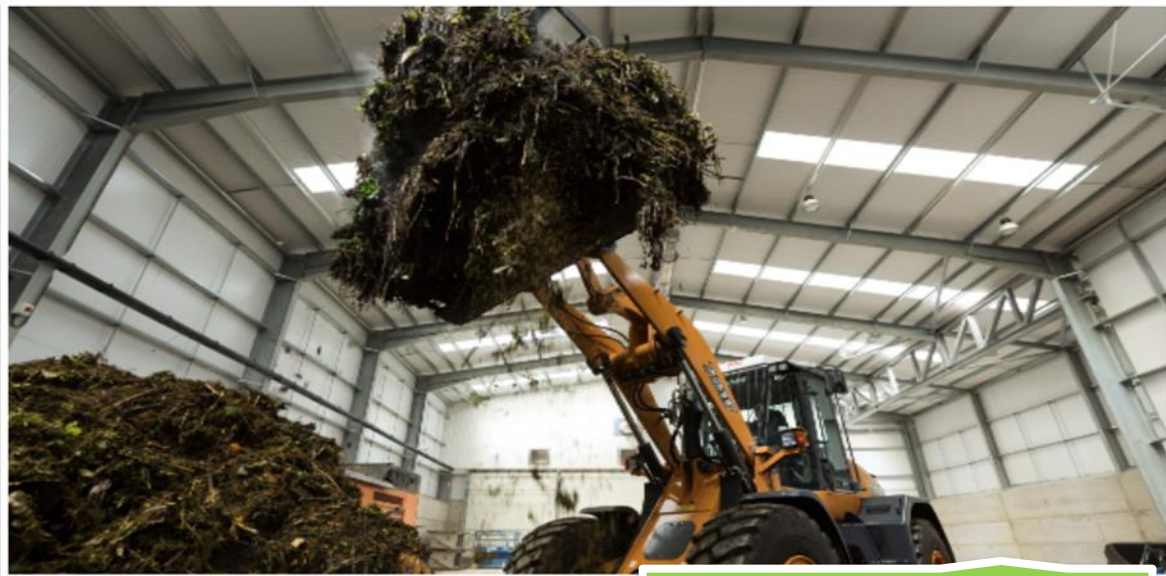
Willerby IVC Facility
