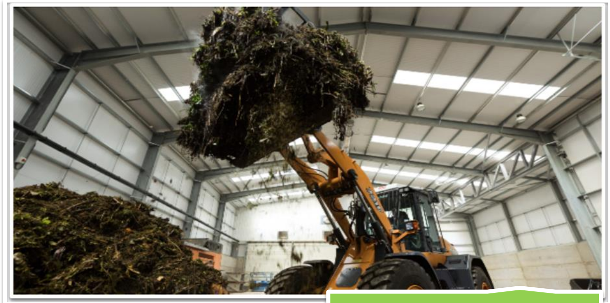
Willerby IVC Facility
