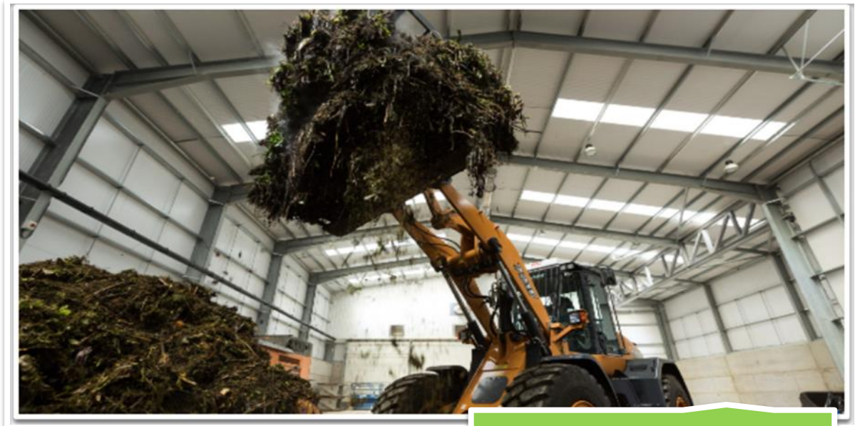
Willerby IVC Facility
