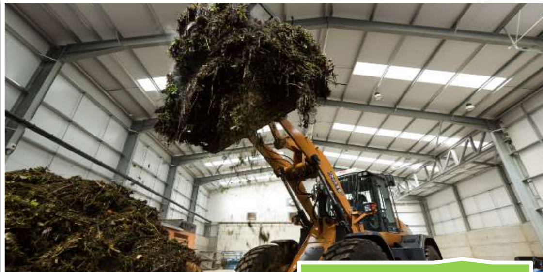
Willerby IVC Facility
