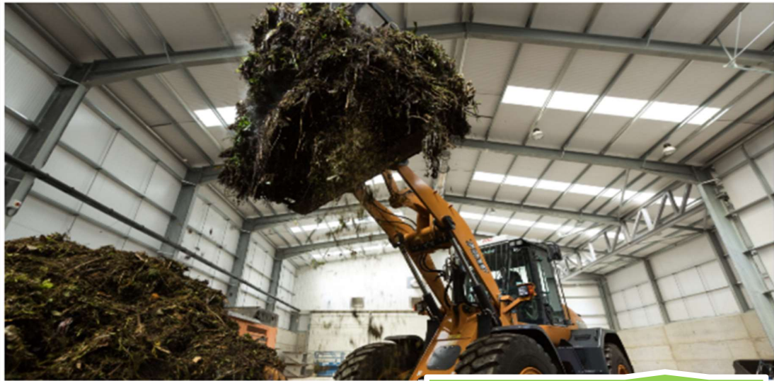
Willerby IVC Facility
