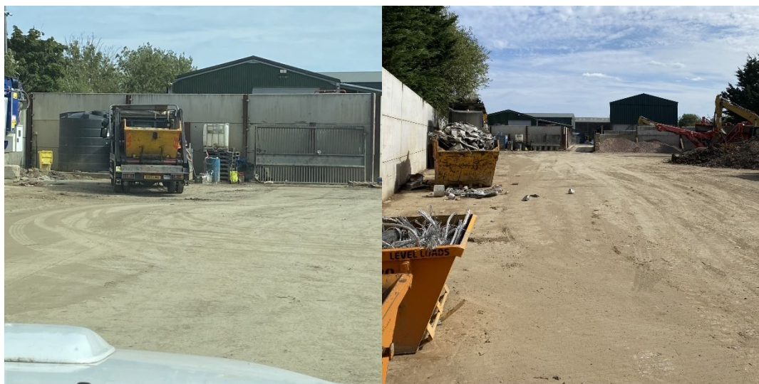
Figure 2. ~3m concrete panelling surrounding site
