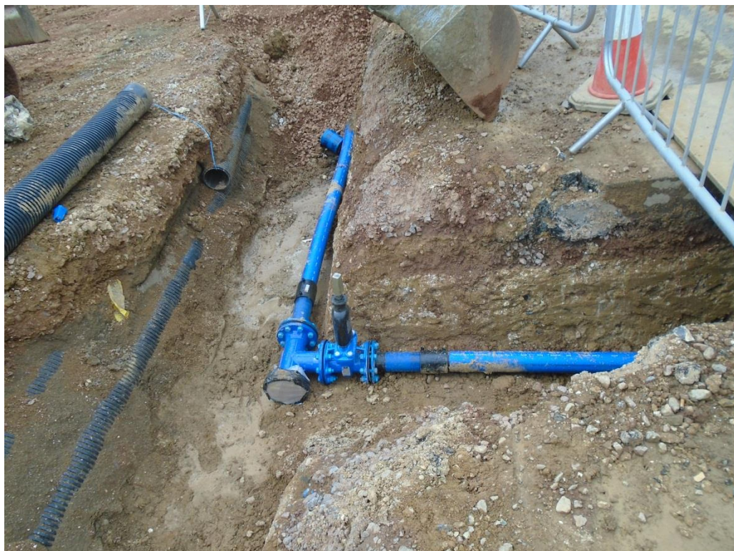
Plate 2 – Installed multi-layer barrier pipe (Protecta-Line)
