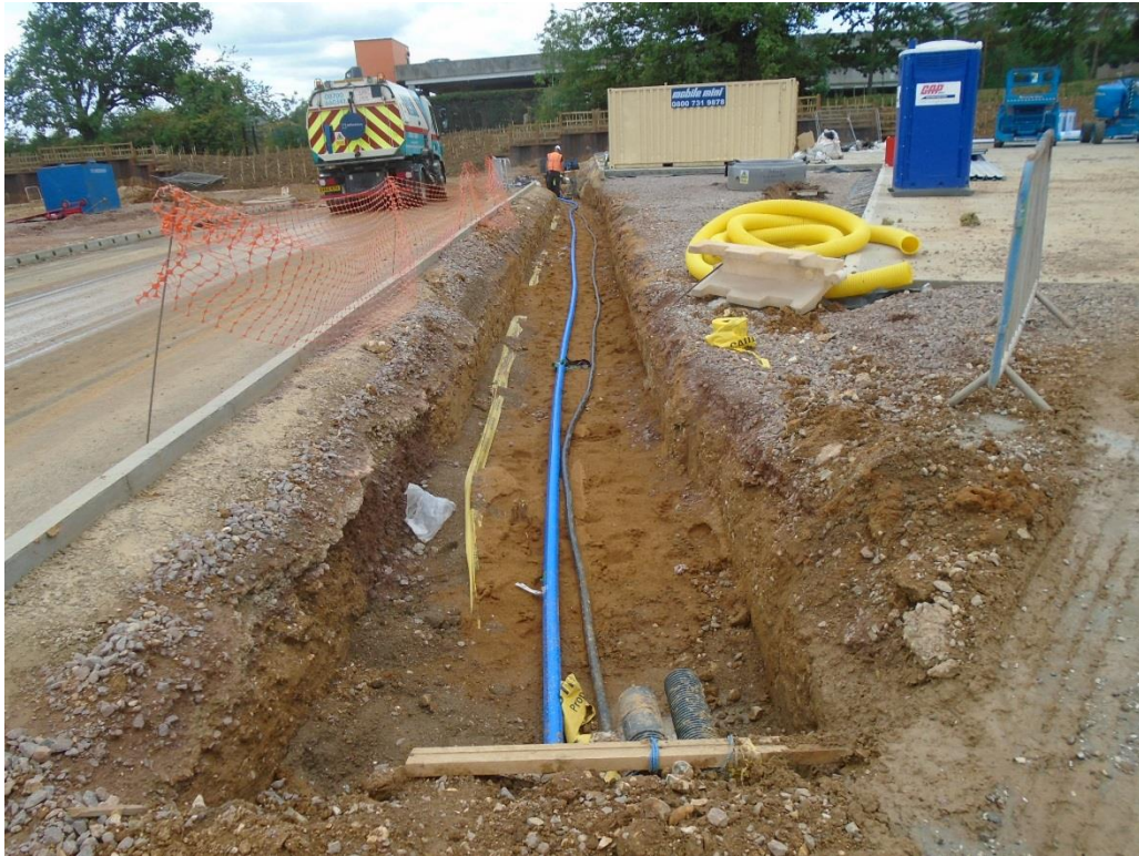
Plate 1 – Installed multi-layer barrier pipe (Protecta-Line)
