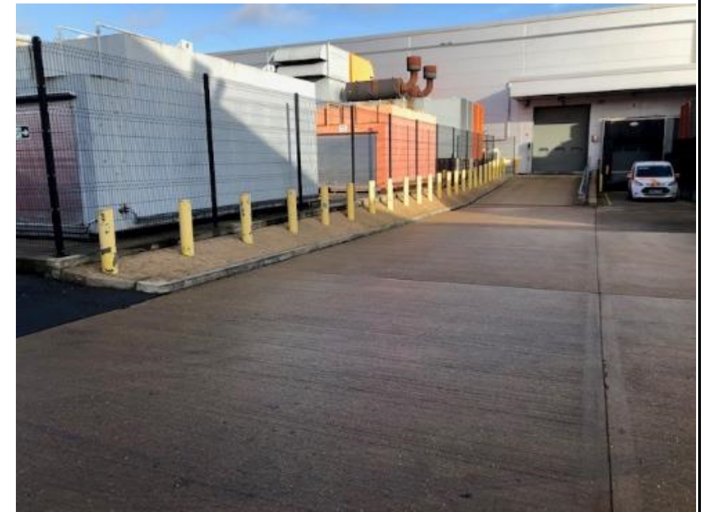
Photo 6: Maylands - Looking north at bulk diesel tanks and towards delivery access route to main building .
