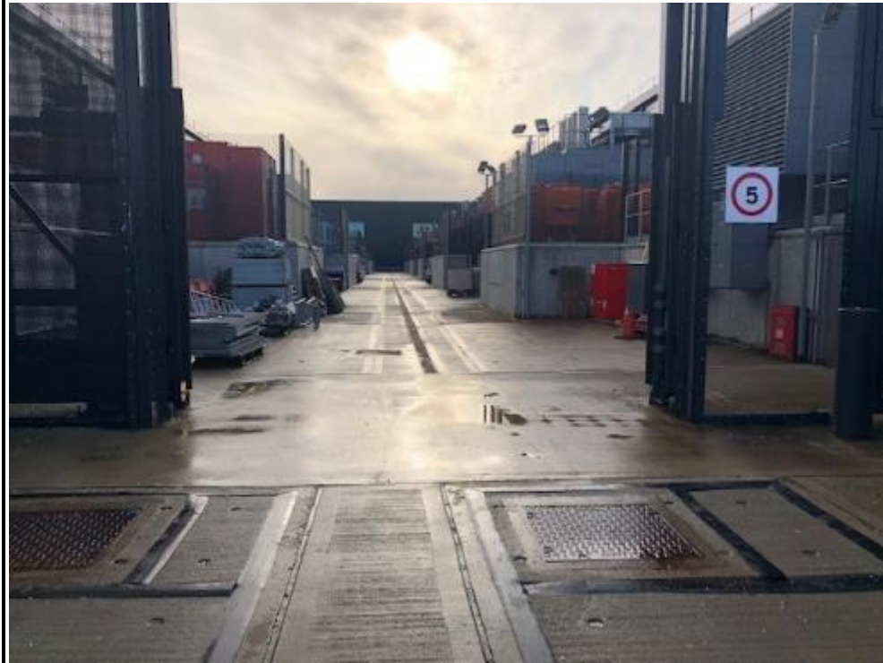
Photo 1: Campus - Entrance to permit area looking south
