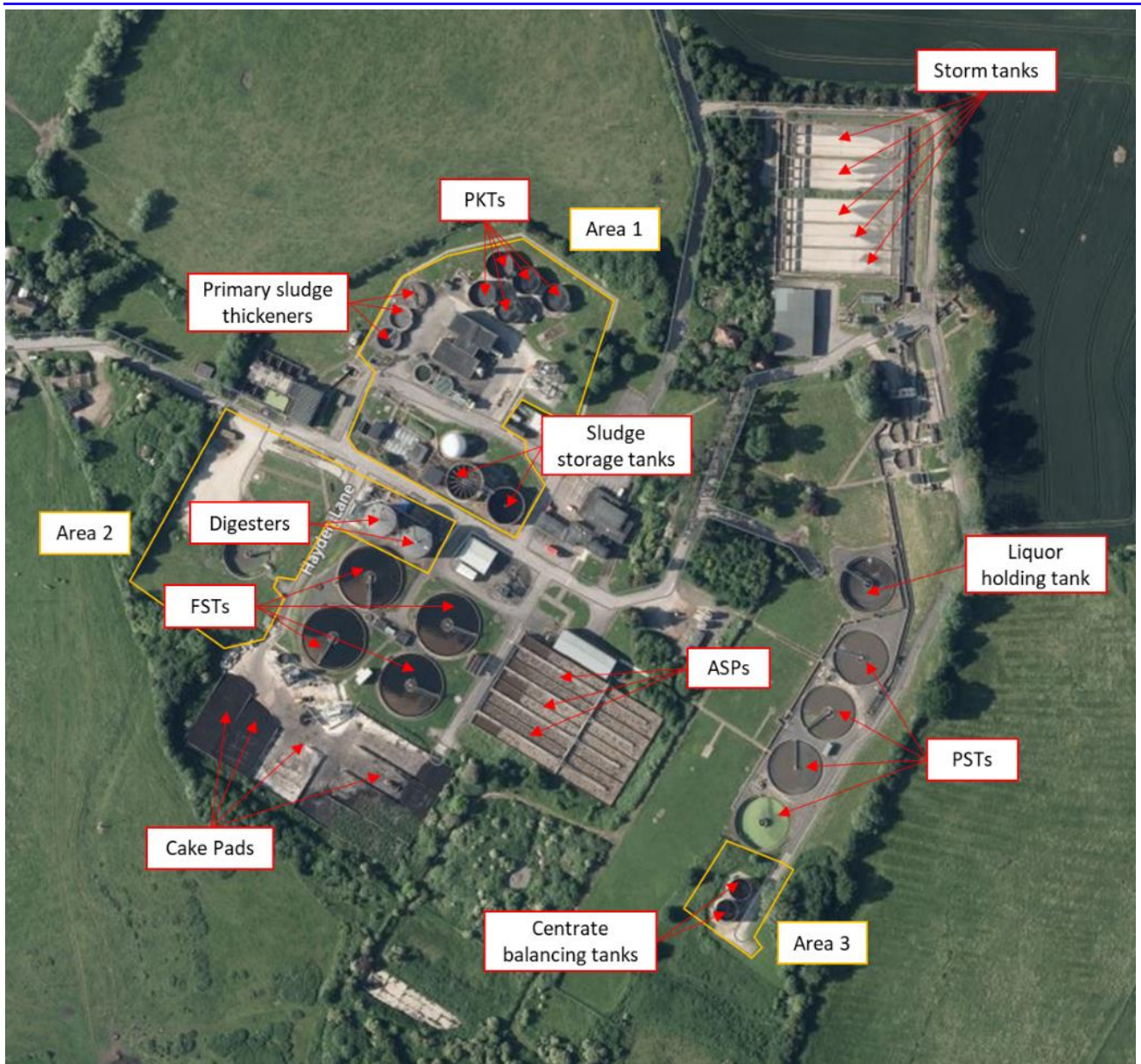
Figure 2.2 Labelled image of Hayden Sewage Treatment Works
