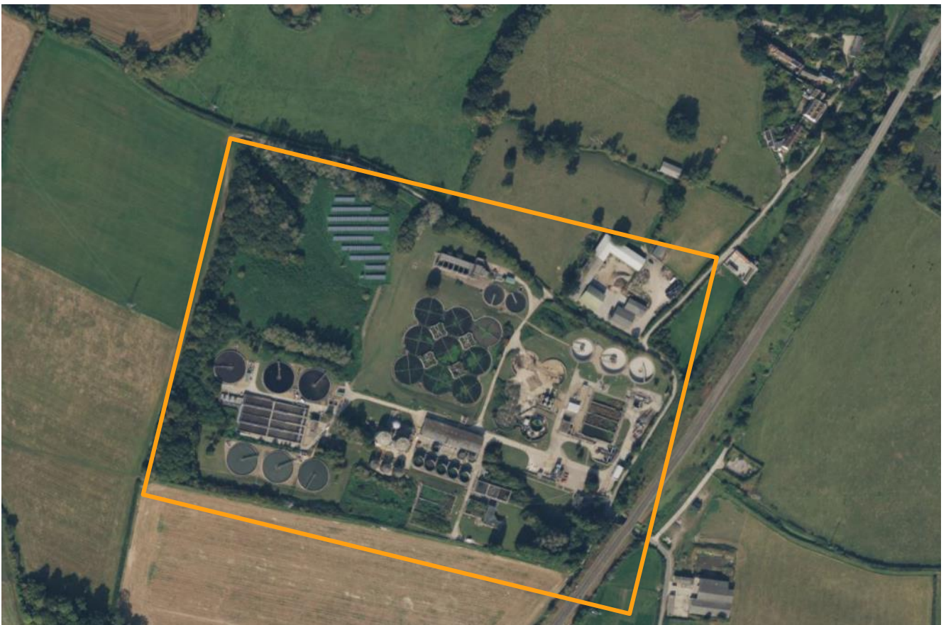
Figure i Satellite view of Stanley Downton Sewage Treatment Works
