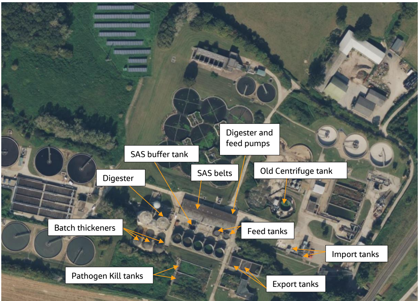
Figure 2.2 Labelled image of Stanley Downton Sewage Treatment Works
