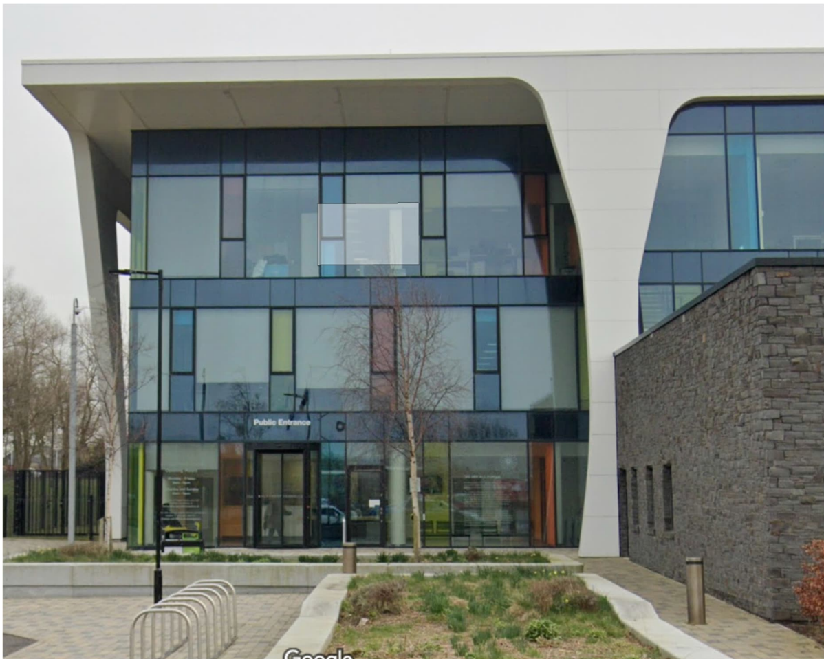
Figure 16 – Blackpool Police Headquarters building
