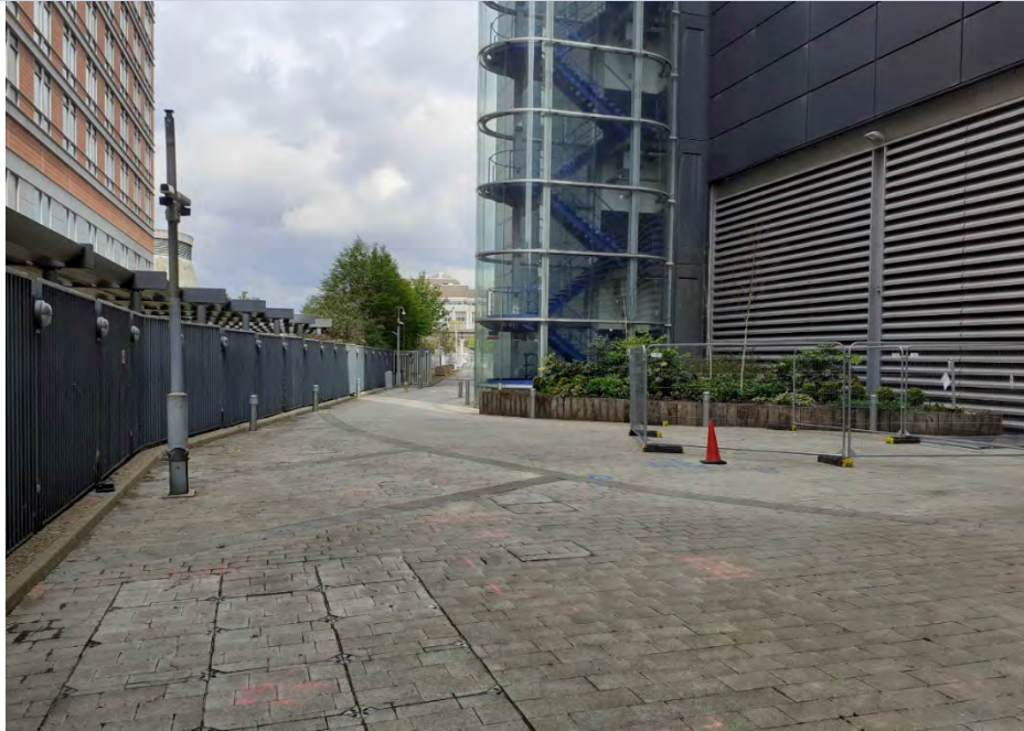
Photo 5 View north across western boundary.
