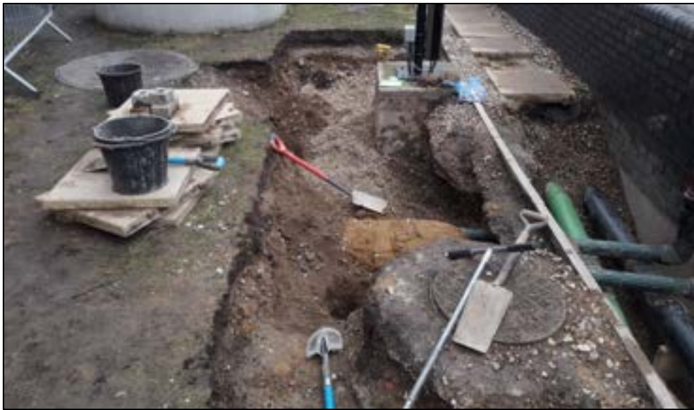
Photograph 6 – Full completed excavation extent (18/02/2021)
