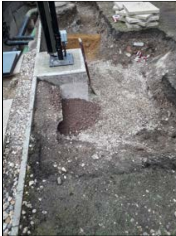
Photograph 9 – Layered backfill of excavation (18/02/2021)
