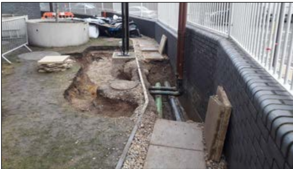
Photograph 7 – Full completed excavation extent (18/02/2021)
