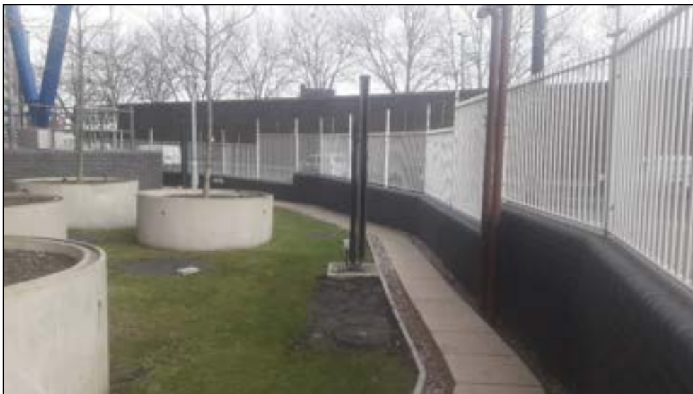
Photograph 1 – Area concerning the point of loss (07/01/2021)
