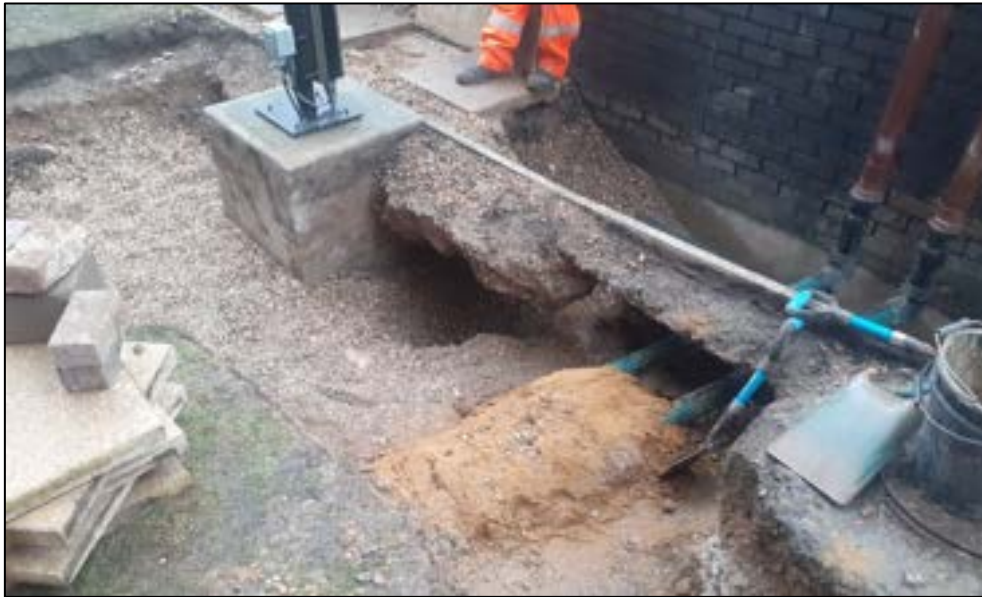
Photograph 8 – Sand over services reinstatement (18/02/2021)
