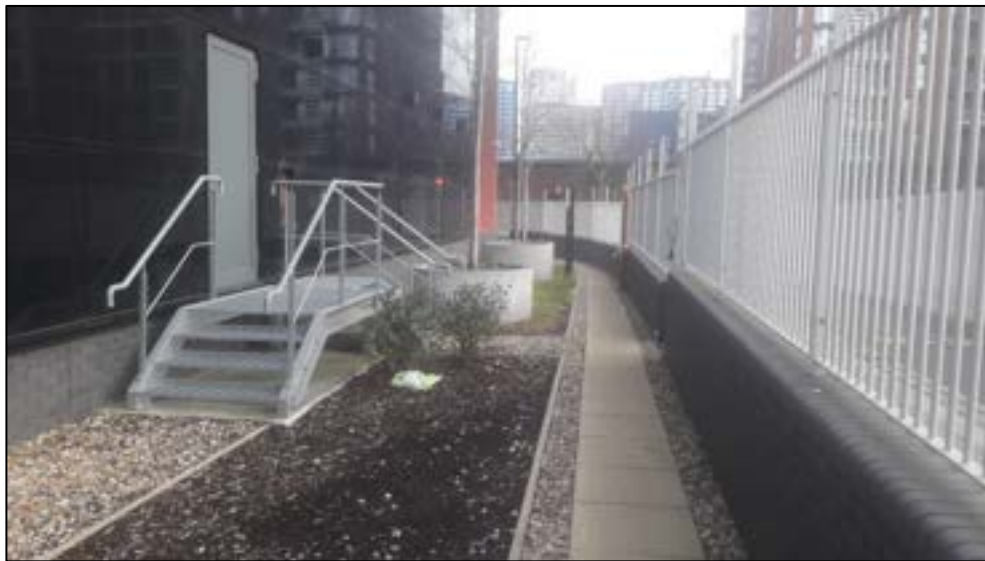
Photograph 2 – Access to point of loss (07/01/2021)
