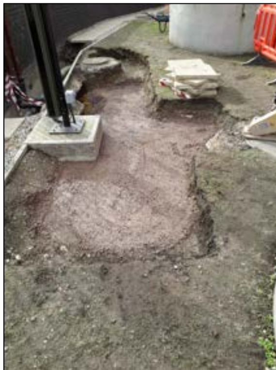
Photograph 10 – Compacted backfill (18/02/2021)
