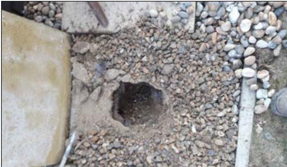
Photograph 4 –Further investigation trial pit on pathway area (11/02/2021)
