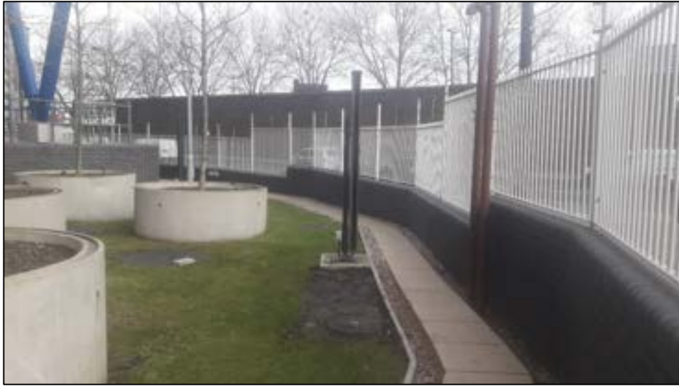
Photograph 1 – Area concerning the point of loss (07/01/2021)
