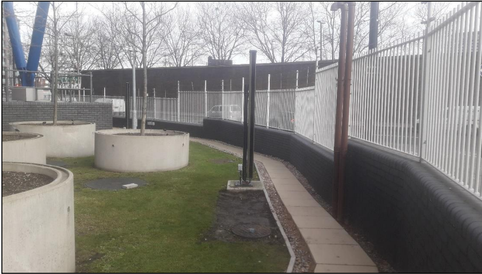
Photograph 1 – Area concerning the point of loss (07/01/2021)
