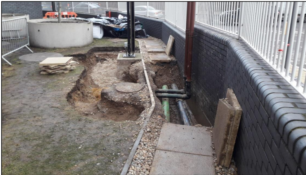
Photograph 7 – Full completed excavation extent (18/02/2021)
