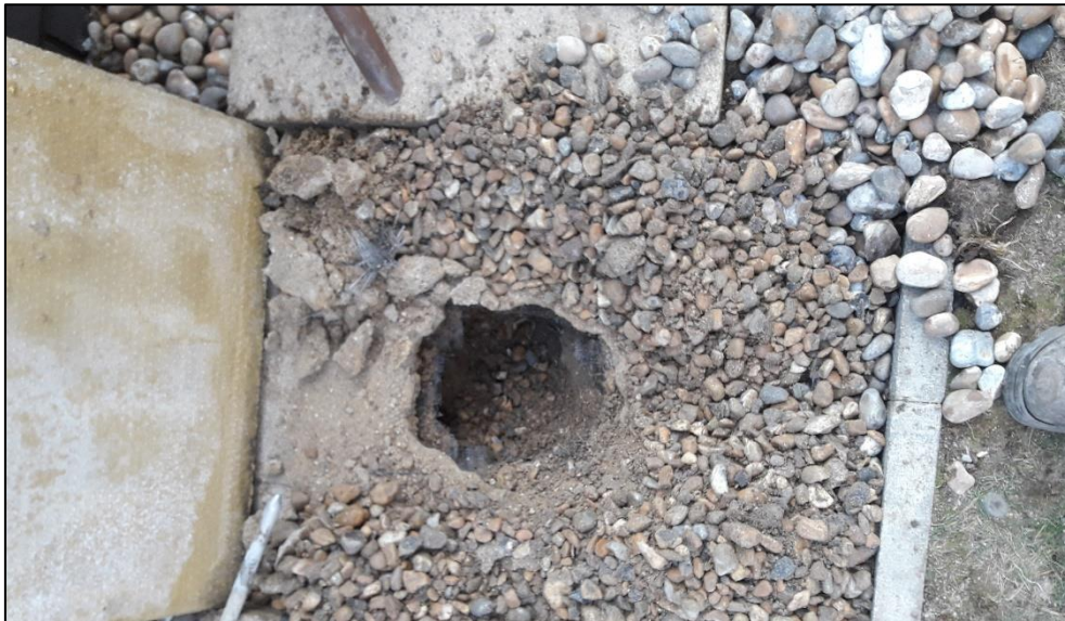
Photograph 4 –Further investigation trial pit on pathway area (11/02/2021)
