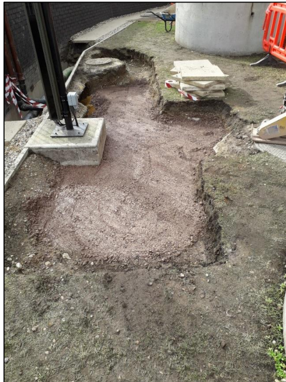
Photograph 10 – Compacted backfill (18/02/2021)
