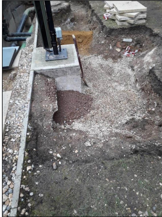
Photograph 9 – Layered backfill of excavation (18/02/2021)
