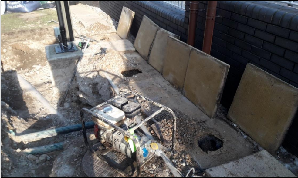
Photograph 5 –Further investigation trial pits (11/02/2021)
