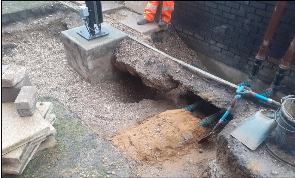
Photograph 8 – Sand over services reinstatement (18/02/2021)
