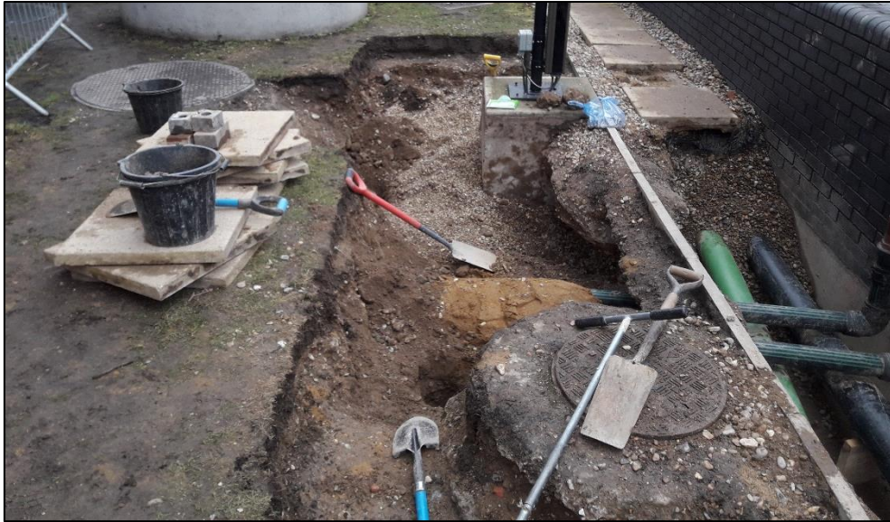
Photograph 6 – Full completed excavation extent (18/02/2021)
