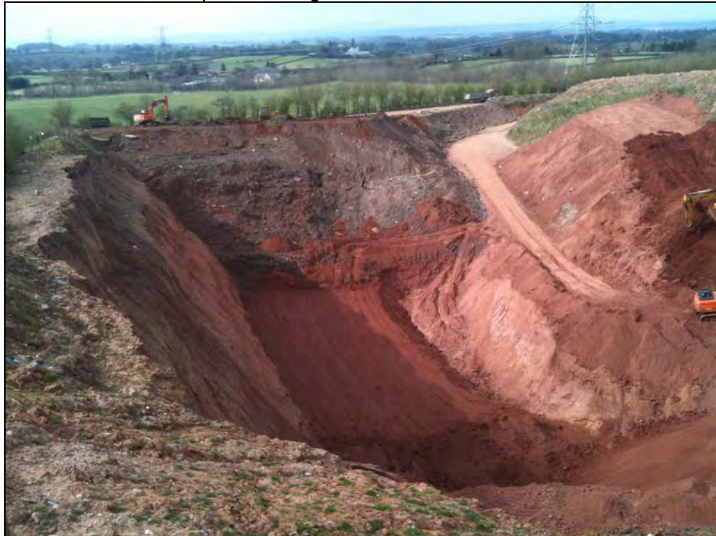
Plate 4:View of completed lining works for Phase 3
