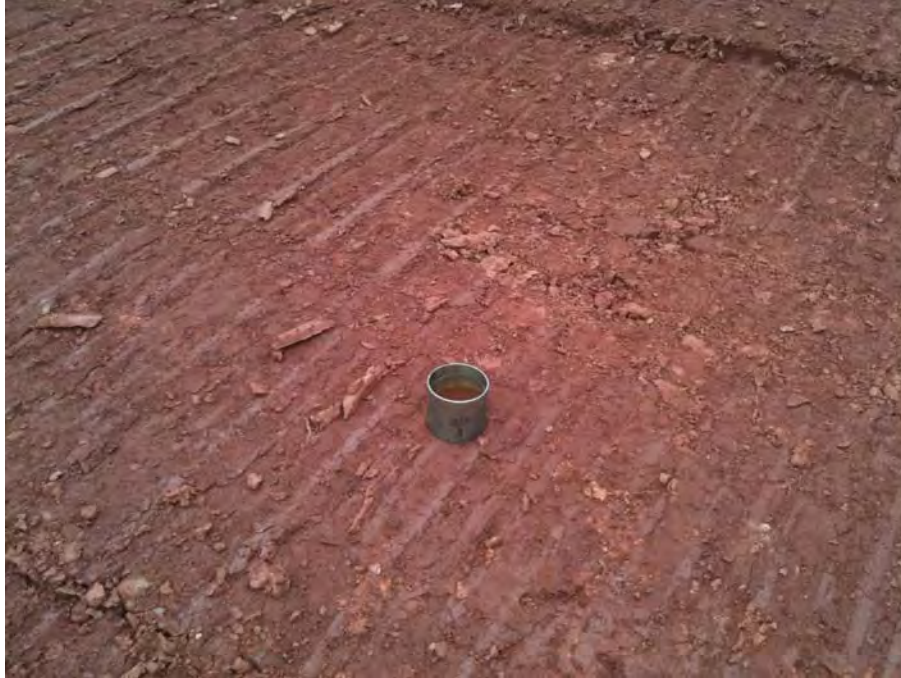
Phase 3 Section 1: Falling Head Permeability 21/03/2011
