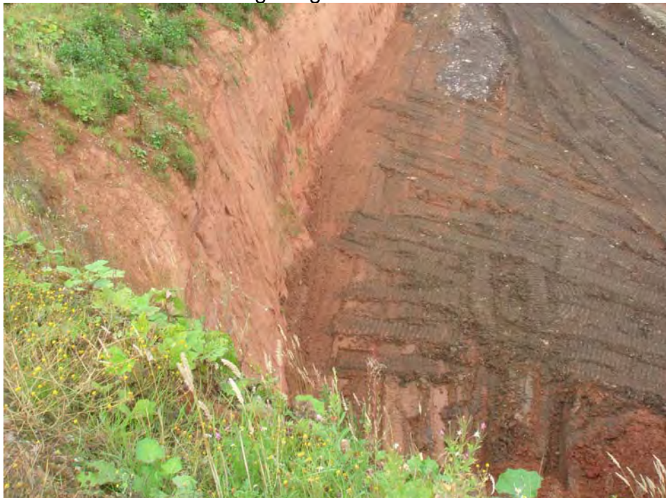
Plate 2: Soil removed off geological barrier
