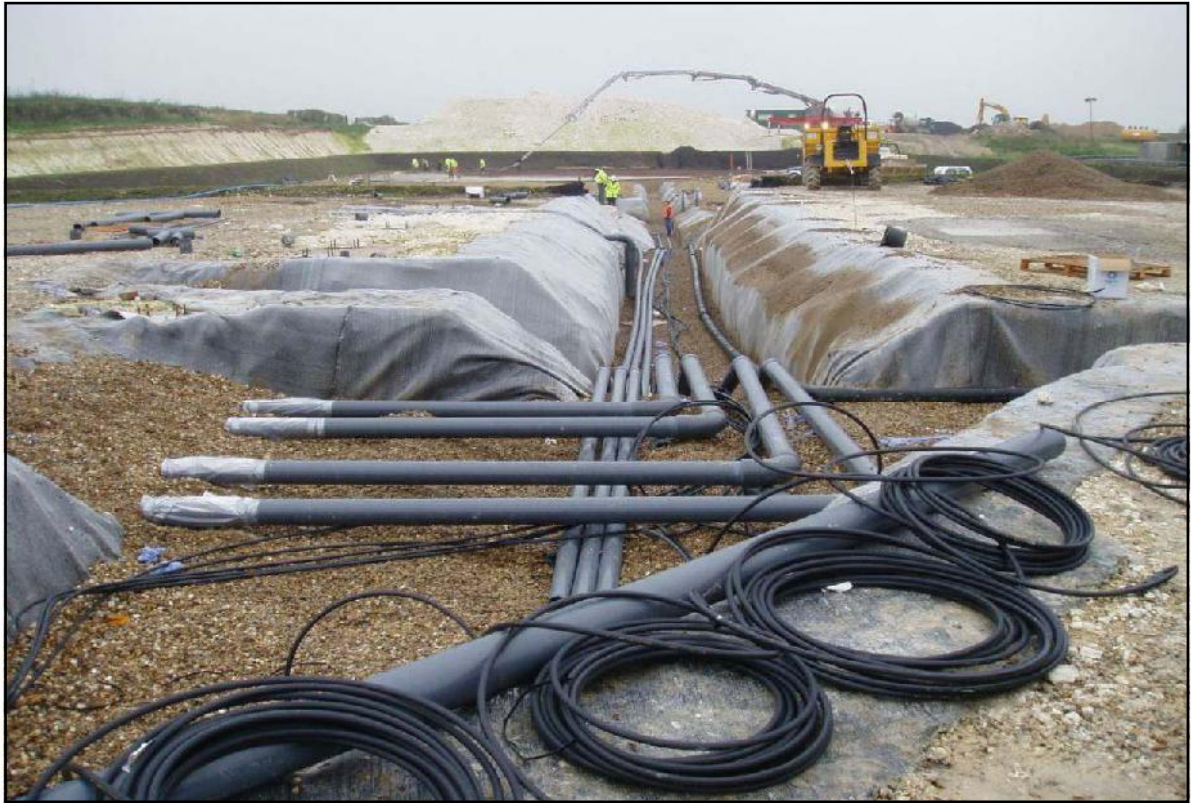
Photo 11. Pipe work installed in GCL lined trench.
