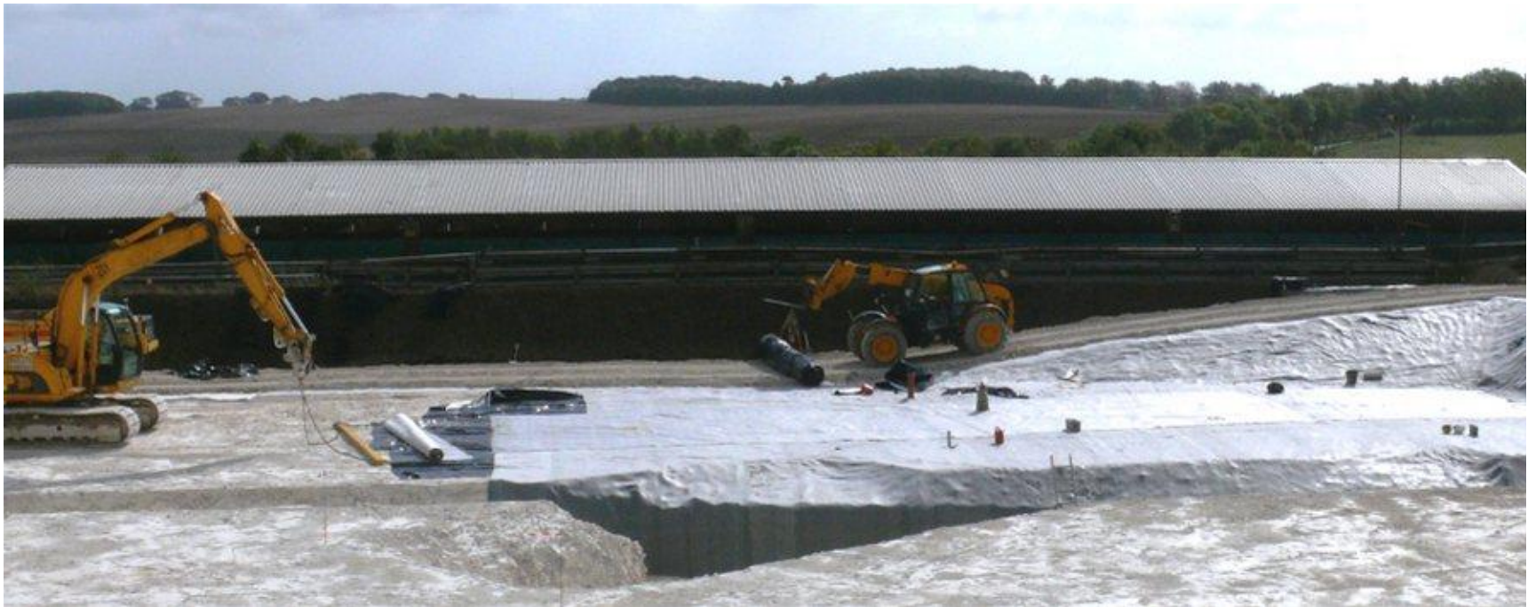
Photograh 3 – Placement of the bentonite liner
