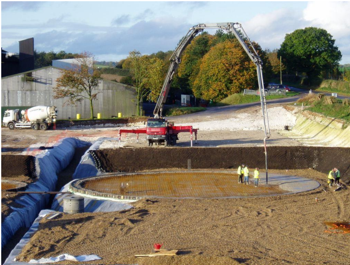
Photograph 8 – Concrete pouring
