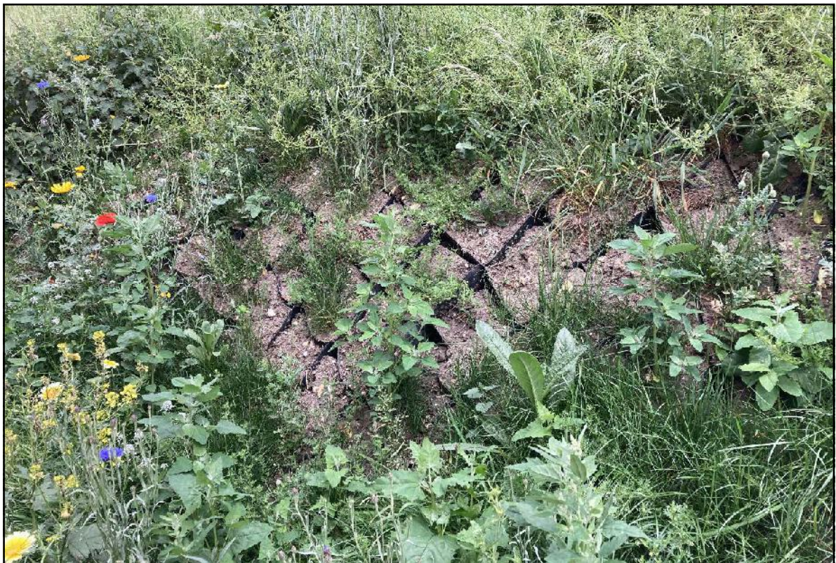
Photo 24. View of eastern margin showing detail of soil-filled EnviroGrid.
