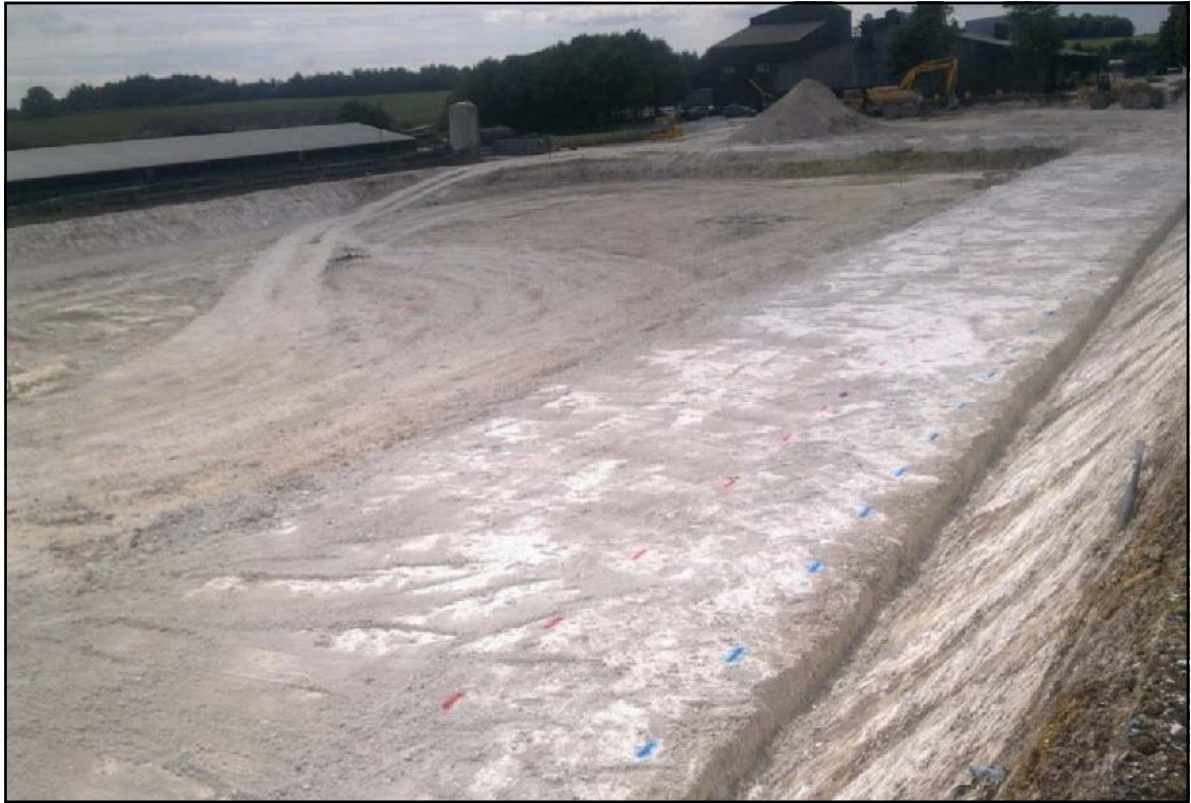
Photo 1. View of chalk excavation looking south - west.
