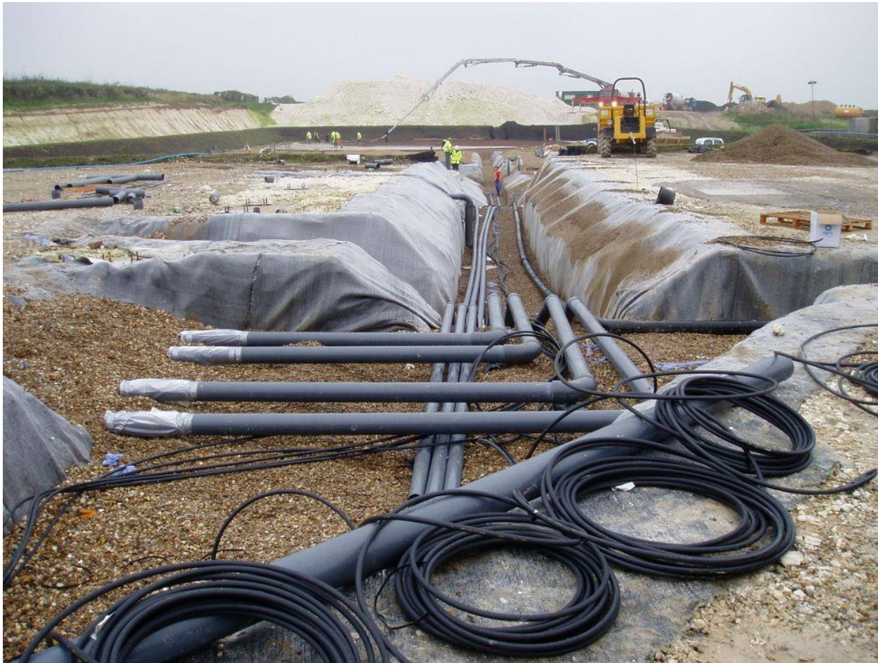
Photograph 12 – Lined trench for pipework
