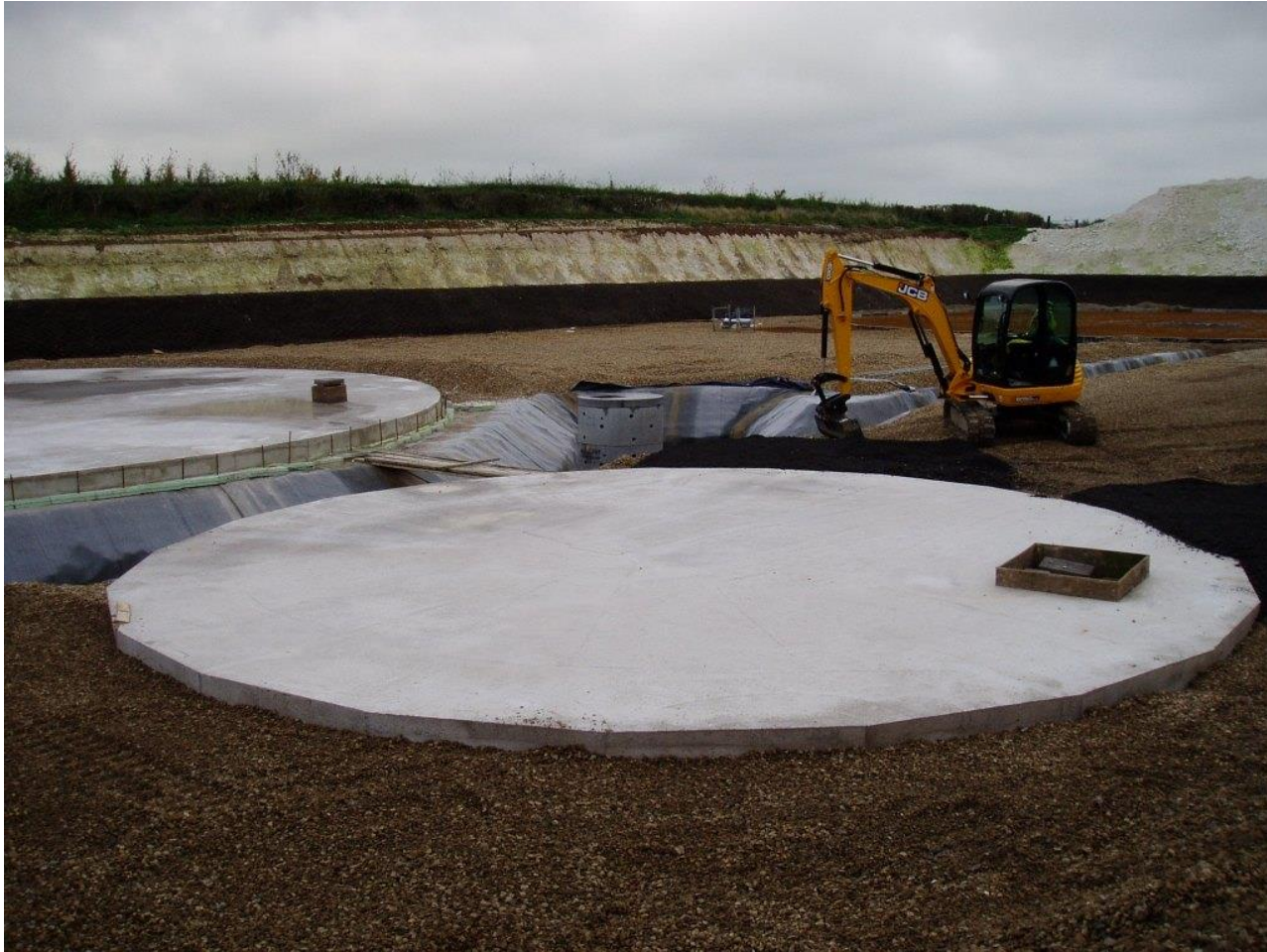
Photograph 11 – Concrete tank bases
