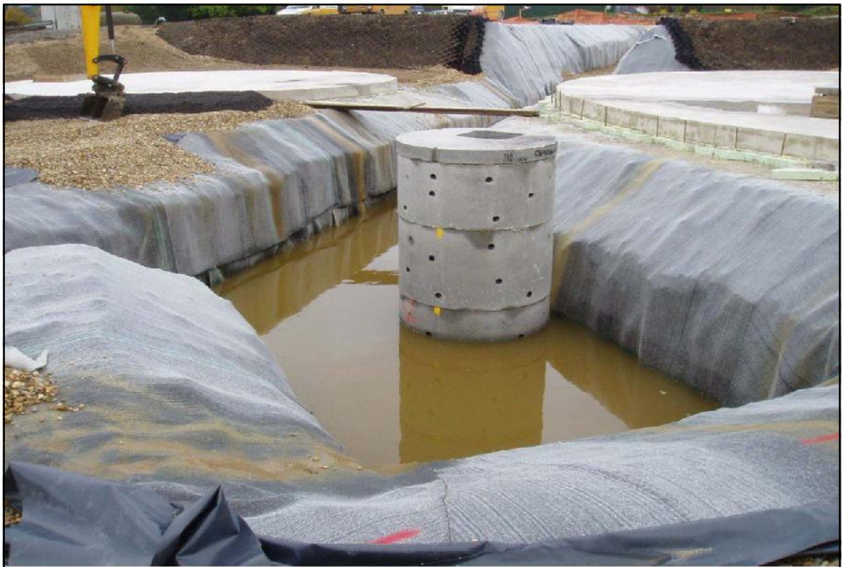
Photo 12. Sump installed in GCL lined trench.
