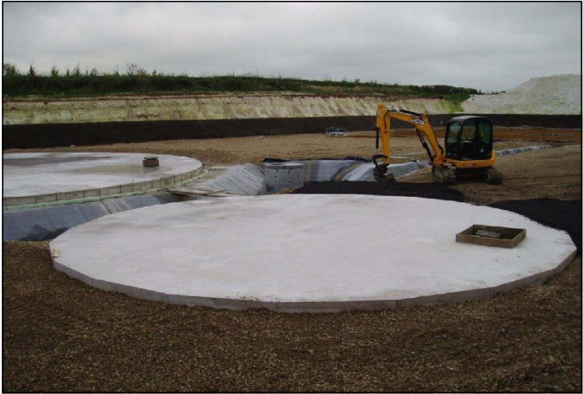
Photo 13. GCL being covered with 300mm clean aggregate..
