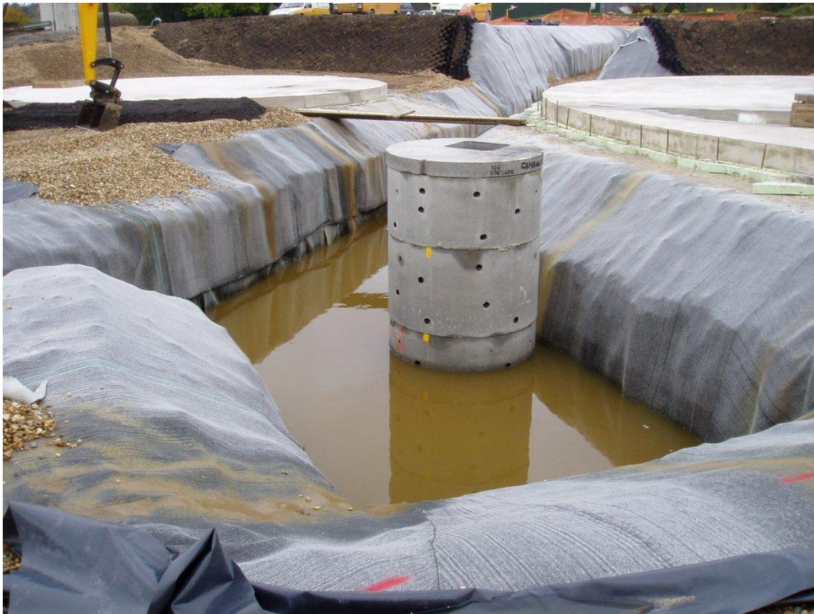
Photograph 10 – Sump within liner
