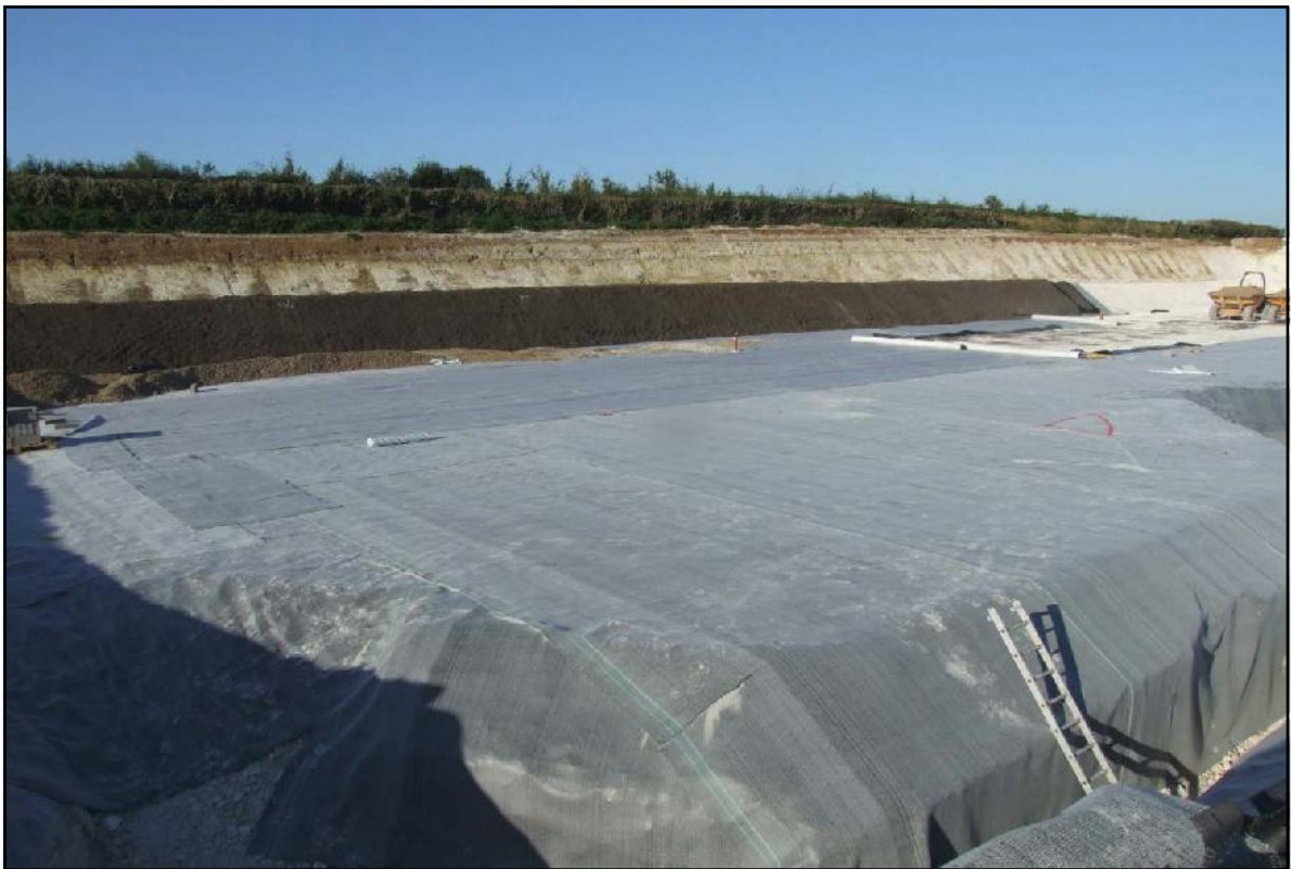
Photo 4. Placement of Geosynthetic Clay Liners (GCL). View looking north.
