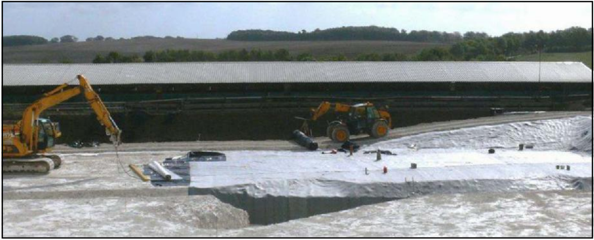
Photo 3. Placement of Geosynthetic Clay Liner (GCL). View looking south.
