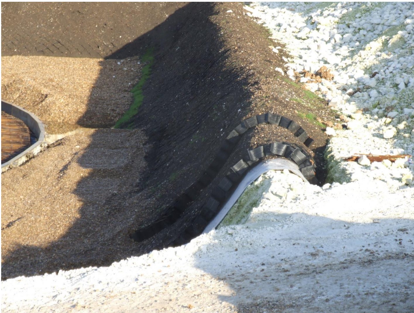
Photograph 5 – Liner secured on side wall using 'Envirogrid'
