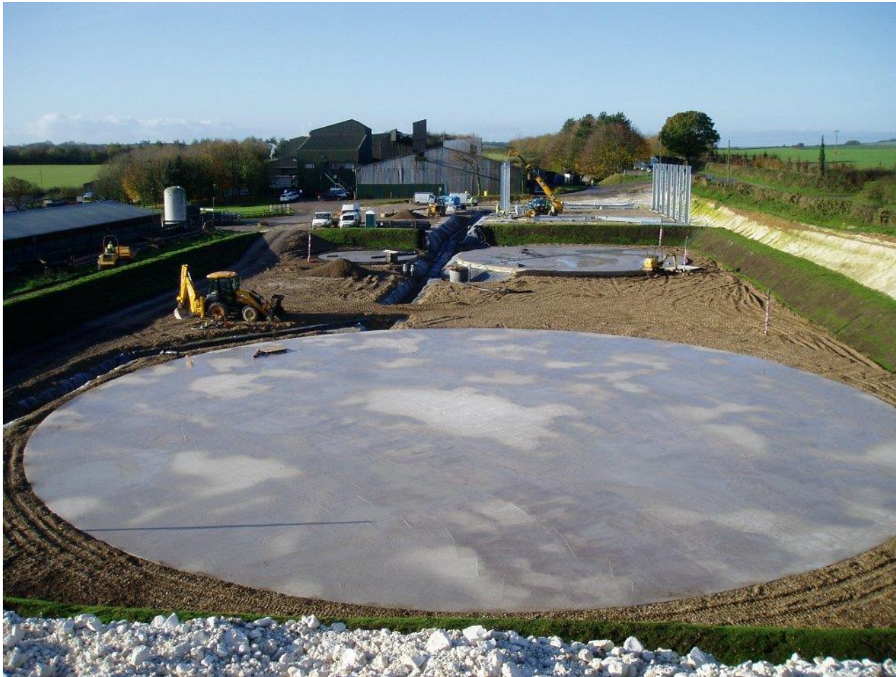
Photograph 13 – Concrete tank bases and grassed banks
