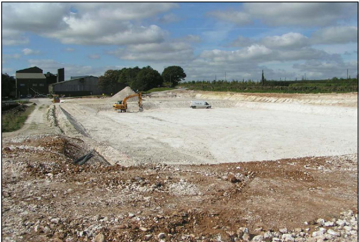
Photo 2. View of chalk excavation looking west.
