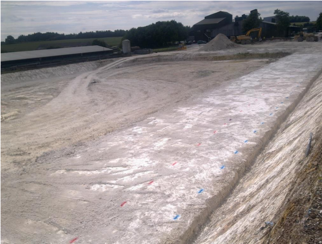
Photograph 1 – Excavation of the chalk
