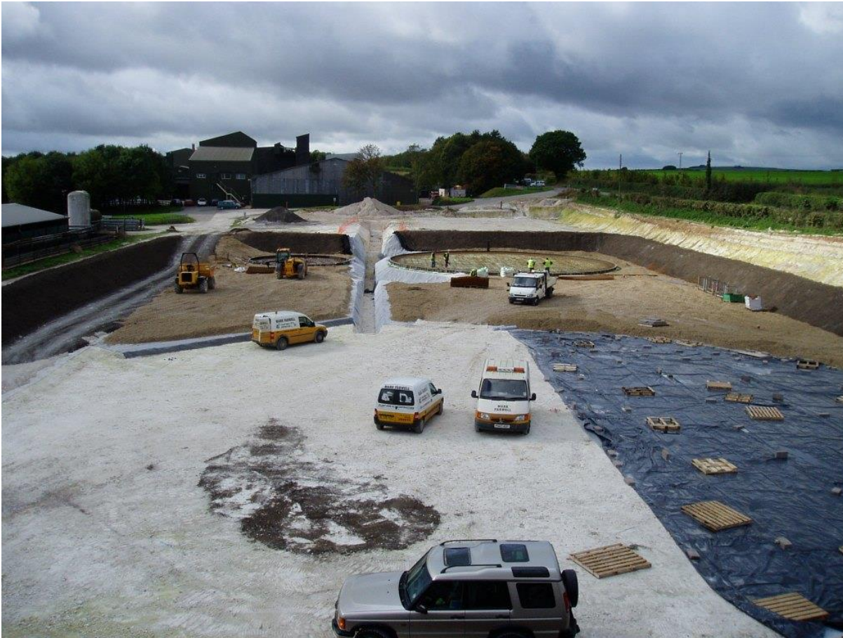
Photograph 2- Excavation and tank bases
