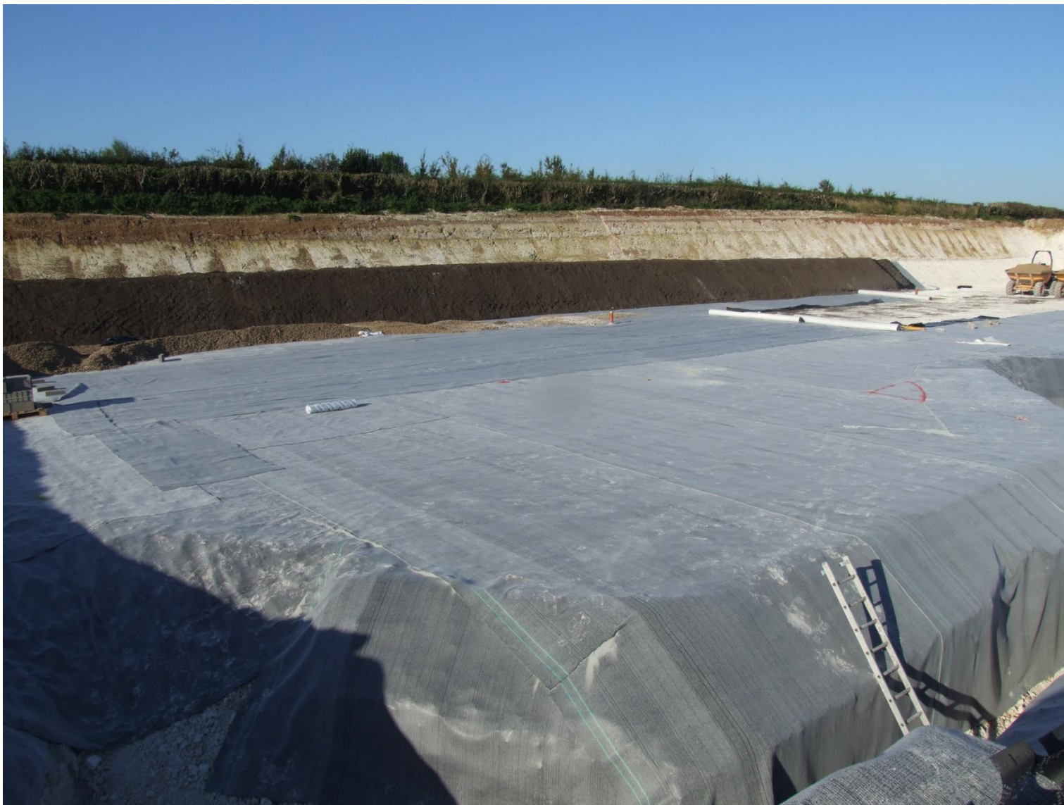
Photograph 4 – Placement of the bentonite liner 2
