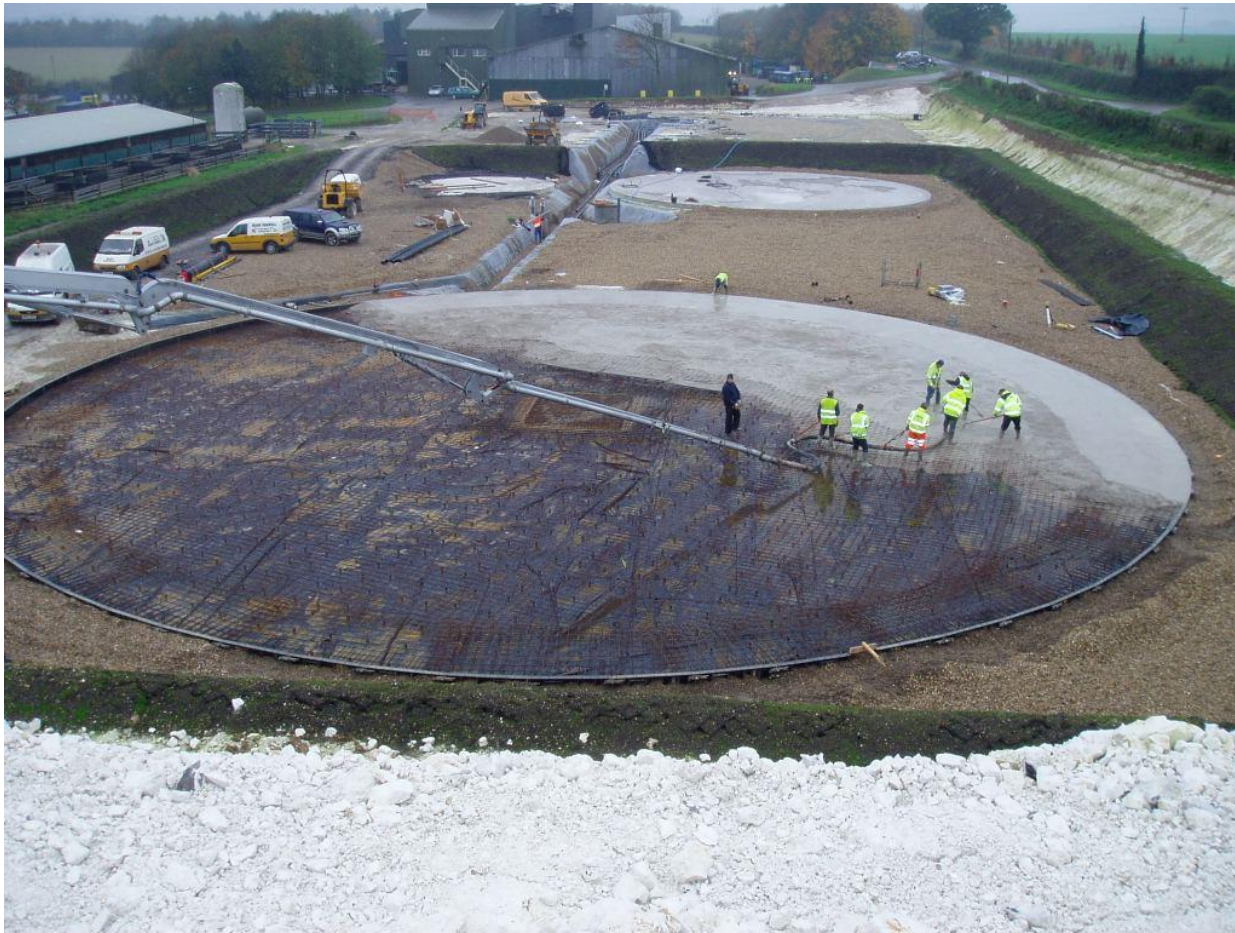
Photograph 11- Site overview during concrete pouring
