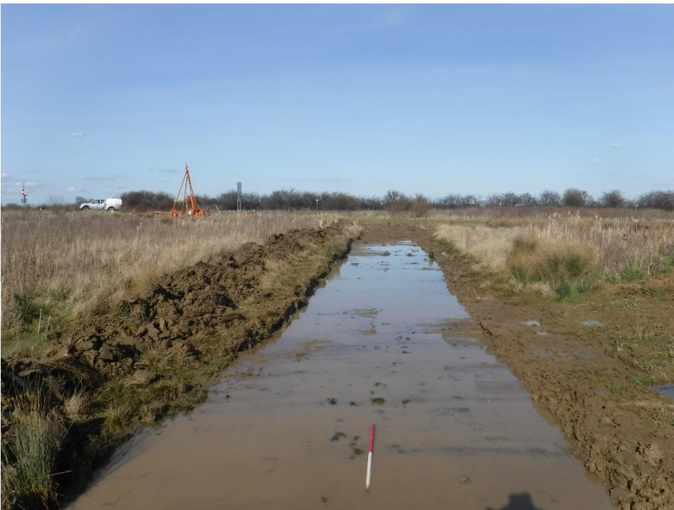
Plate 12: Trackway 1, facing northeast
