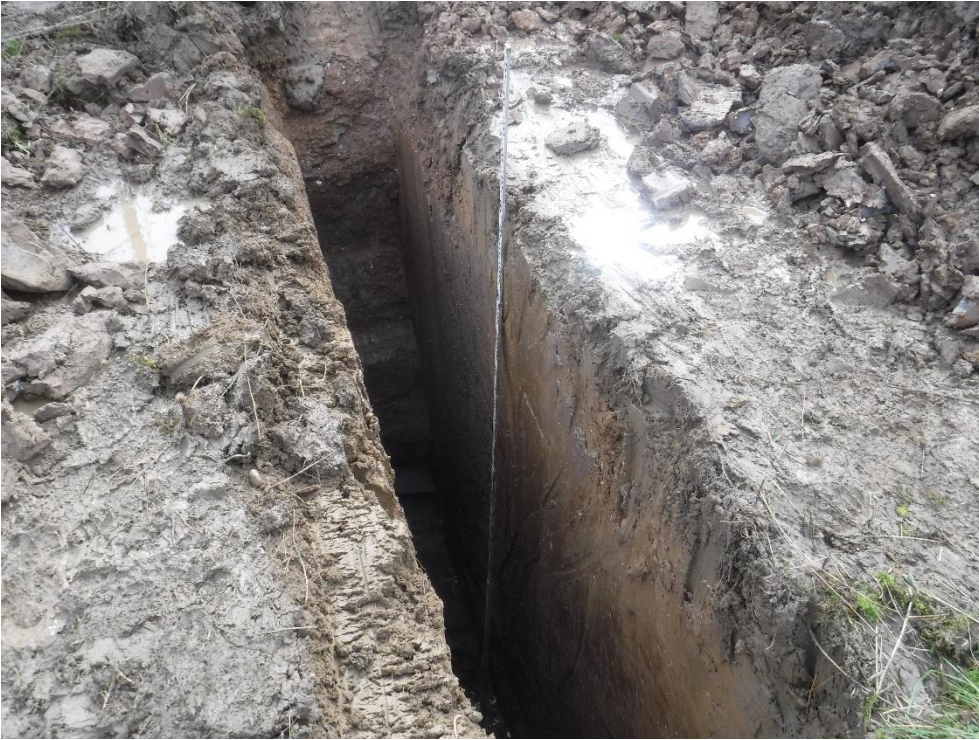
Plate 5: Test Pit 8, facing north
