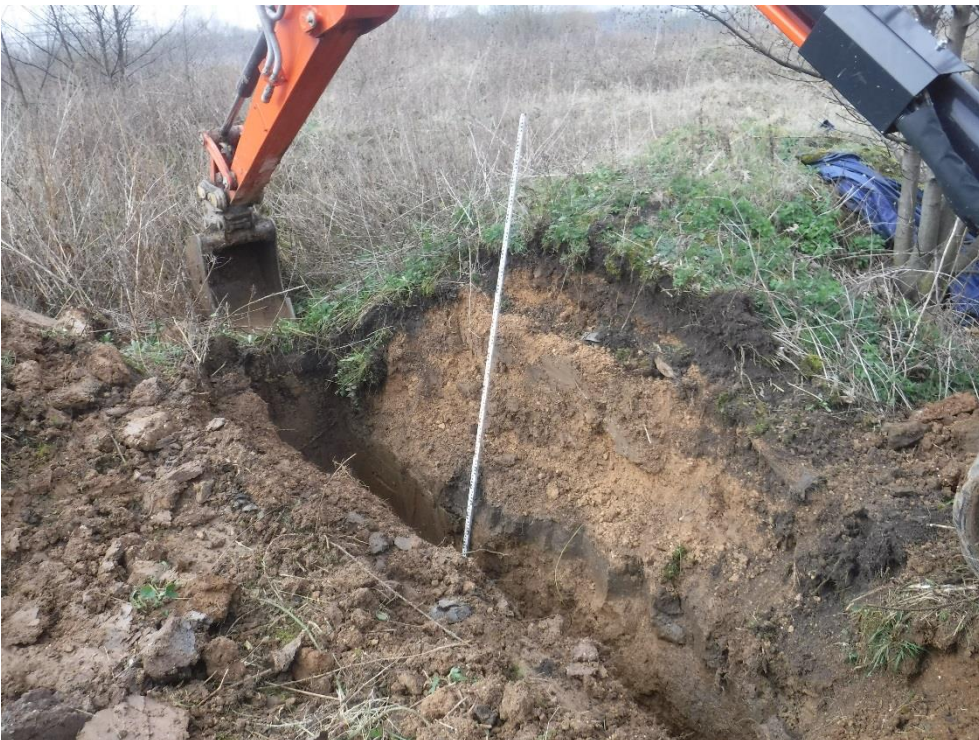
Plate 6: Test Pit 9, facing northwest
