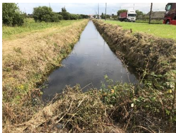
Photo 4 View downstream towards the Port of Immingham (TA1738316736) at 14:21 on 26/07/2023 (on the ebb tide)
