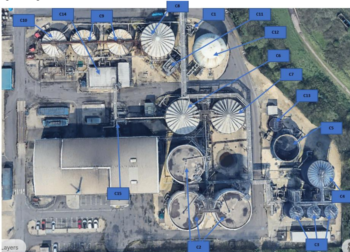
Figure 9 Digester & HPH Area
