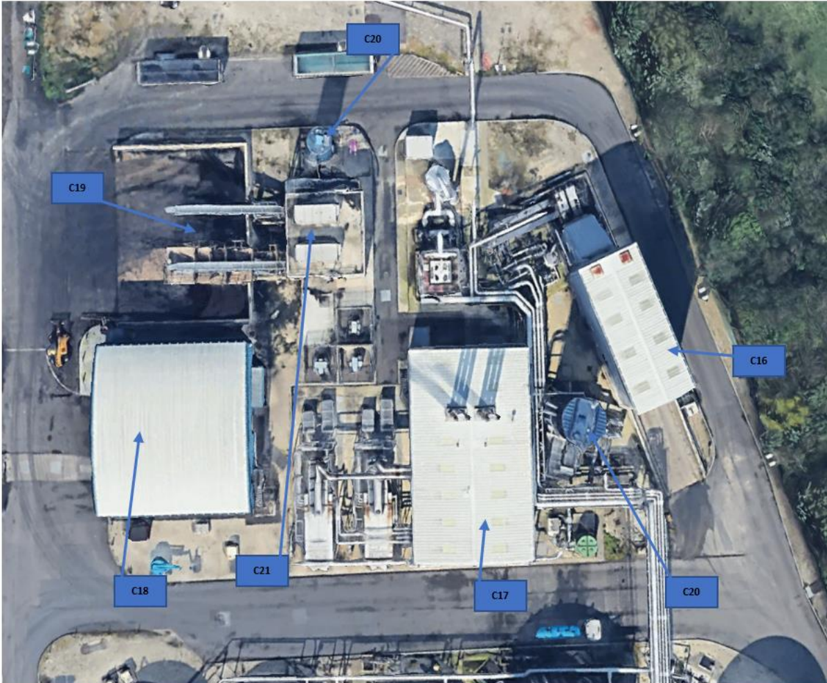
Figure 10 Boiler House & Cake Reception Area:
