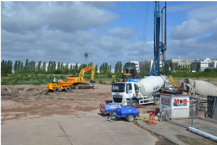
Photo 1: Construction plant operating during A-site works
