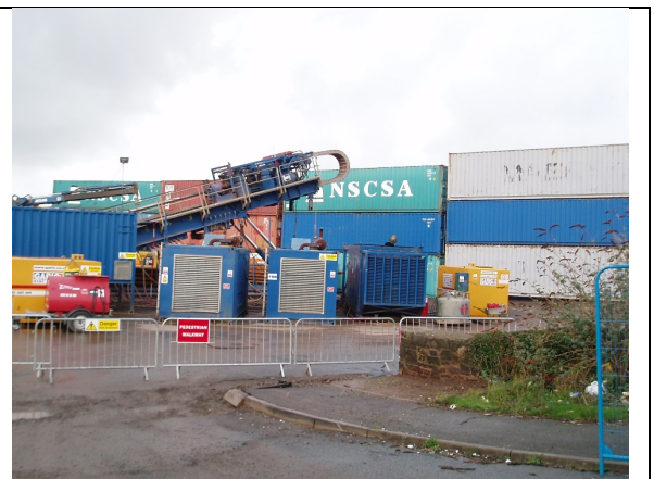
Photo 4: Noise barrier construction from ISO shipping containers
