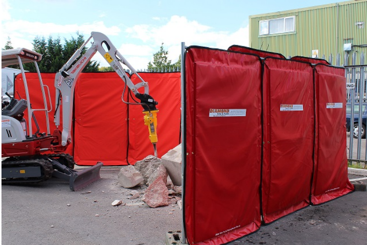
Photo 2: Portable acoustic screen installed around a specific noisy activity.
