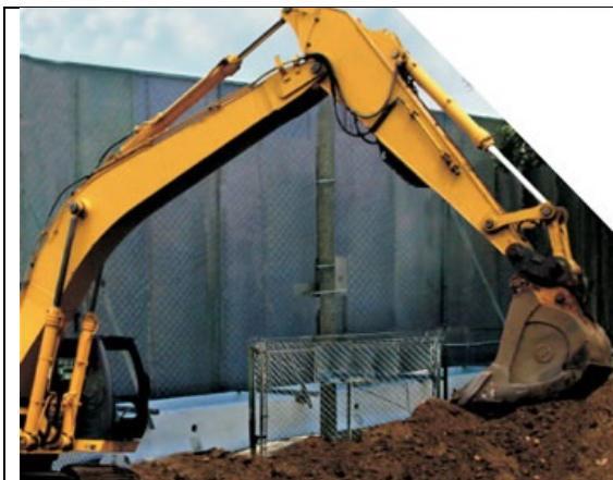
Photo 3: Noise barrier construction from individual mats, attached to support frame.
