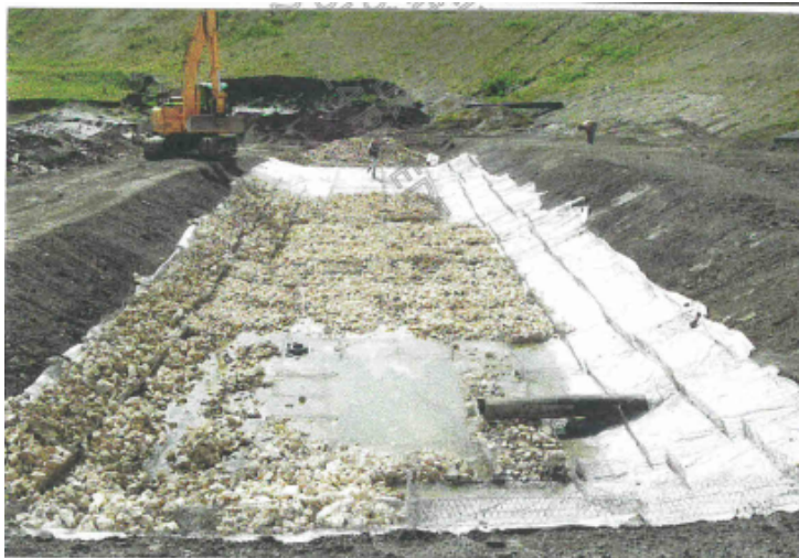
Figure 3-A - Construction of the lagoon and intake pipe protection 4
