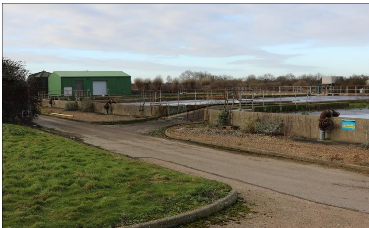
Figure 16. Emergency sludge storage tanks 3 & 4.
