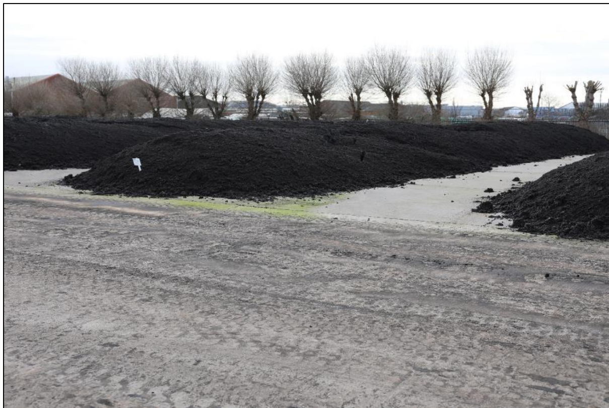
Figure 18. Sludge cake storage pad.
