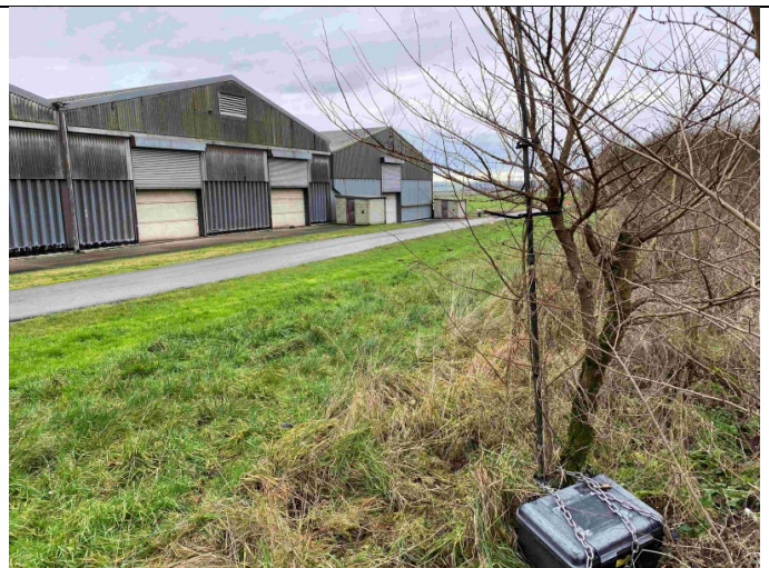
NML1 monitor adjoining farm sheds with grain dryers
