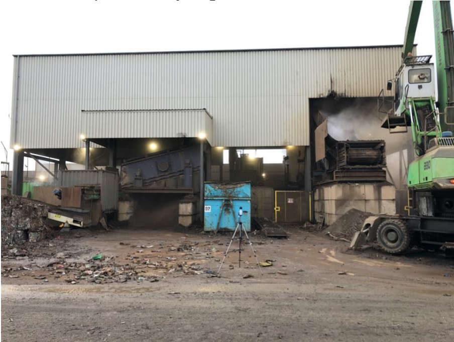
Figure B 1: Sennebogen 830E telehandler operational at the shredder.
