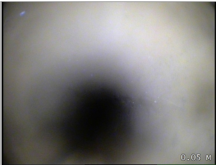
Start node type, manhole, reference s4
