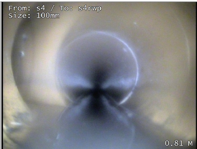
Junction at 9 o'clock, diameter 100mm
