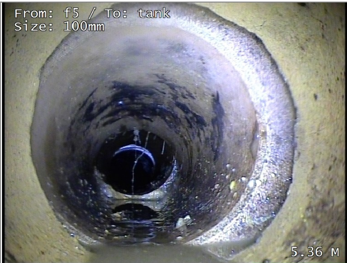
Open joint large
