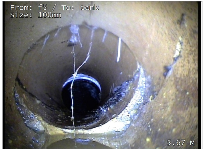
Open joint large
