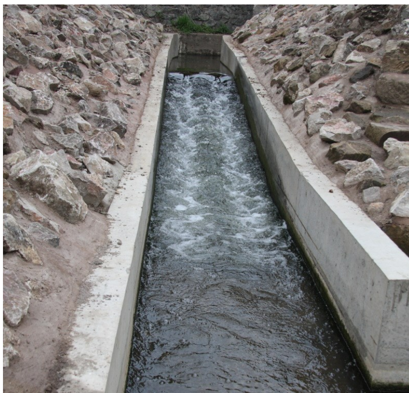
Figure 8.2: Image of an operational Larinier fish pass, showing the highly turbulent flow in the pass.
