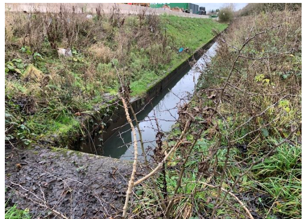
Figure 2.7: Culvert and waterway
