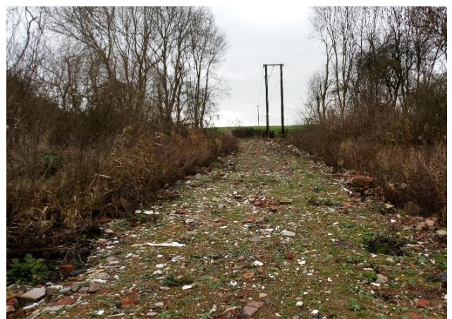
Figure 2.9: Electricity cables through the northwest of the site buried with what looks to be Made Ground
