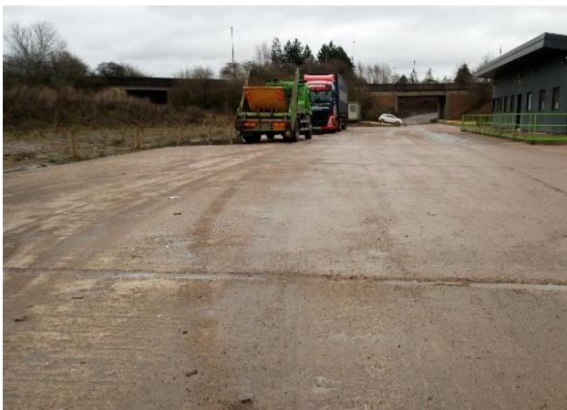
Figure 2.6: Entrance to adjacent site and access road to the proposed development
