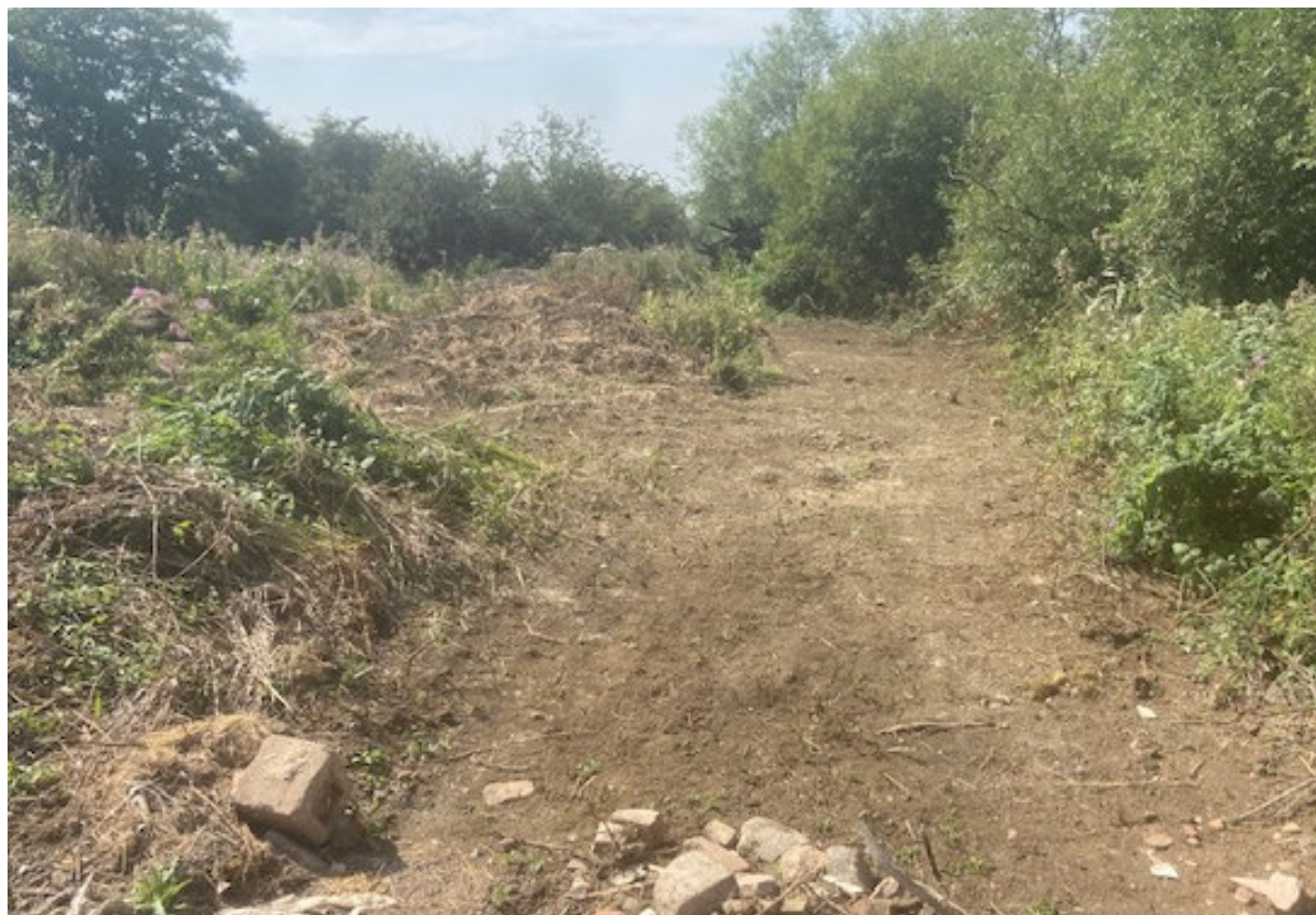
Photograph 2 – Clear vegetated area to access exploratory holes to the west of site.
