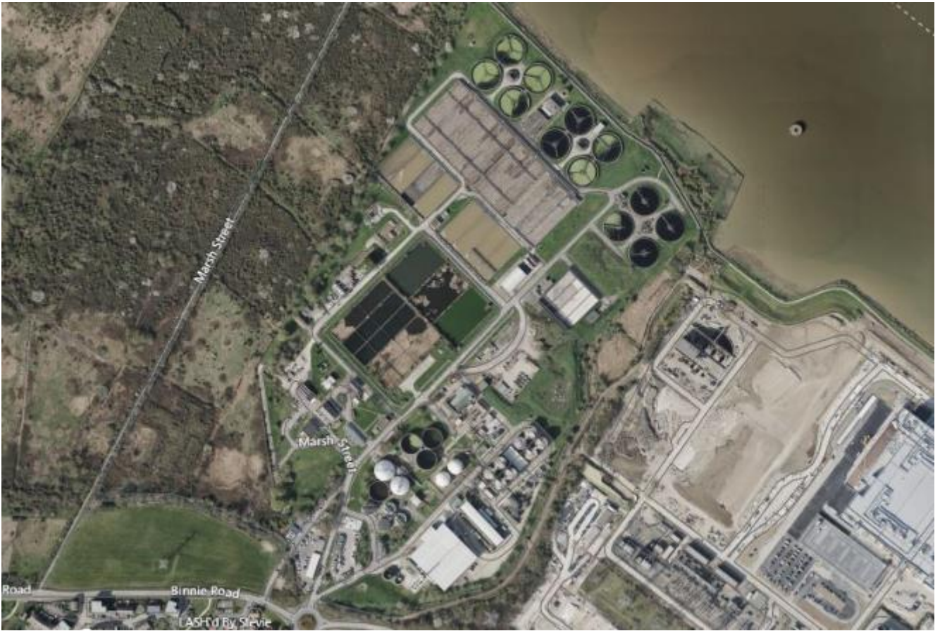
Figure ii Satellite view of Long Reach Sewage Treatment Works and STC
