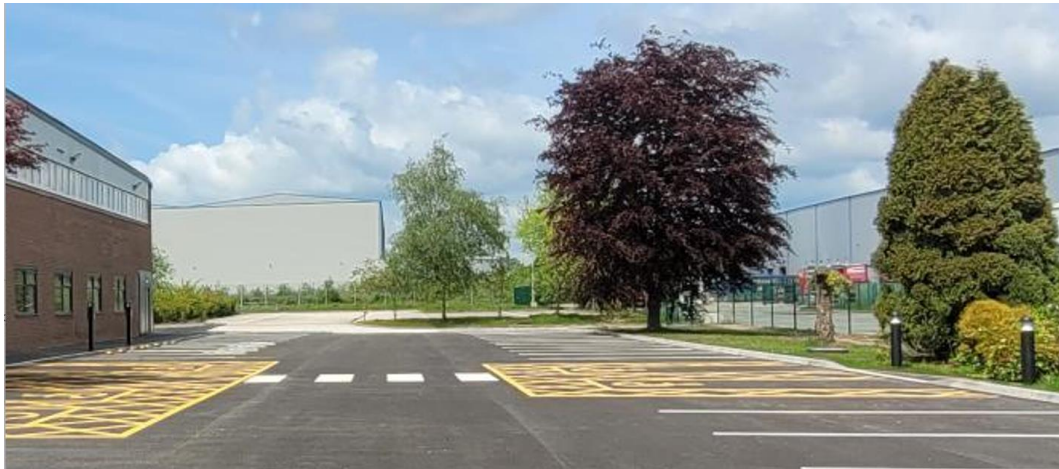
Figure 5 – Looking Towards the Northeast Corner of the Site
