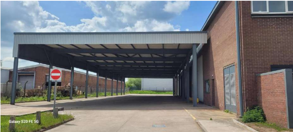
Plate 4 External Storage Area on South Side of Building
