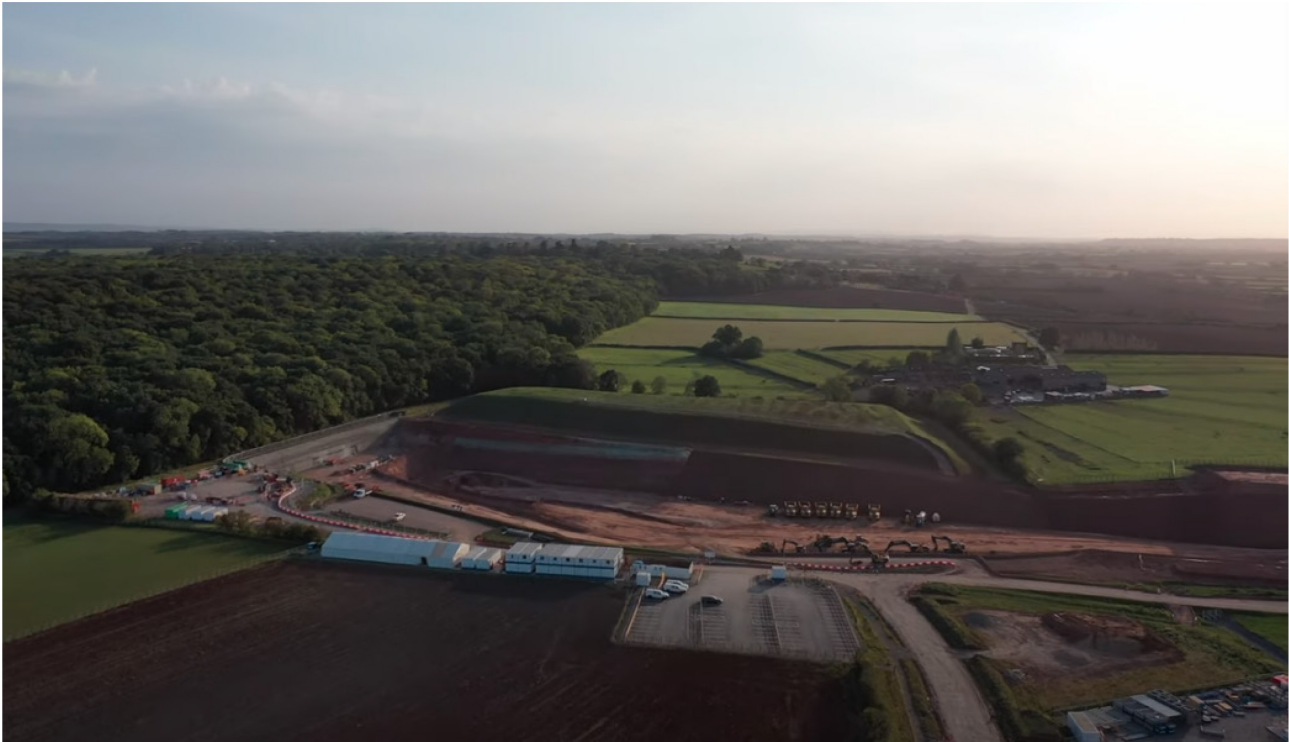
Figure 1.1 Long Itchington Wood North Portal site
