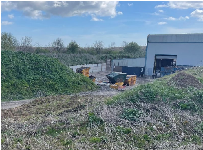
Figure 1: Photograph of bund and retaining wall
