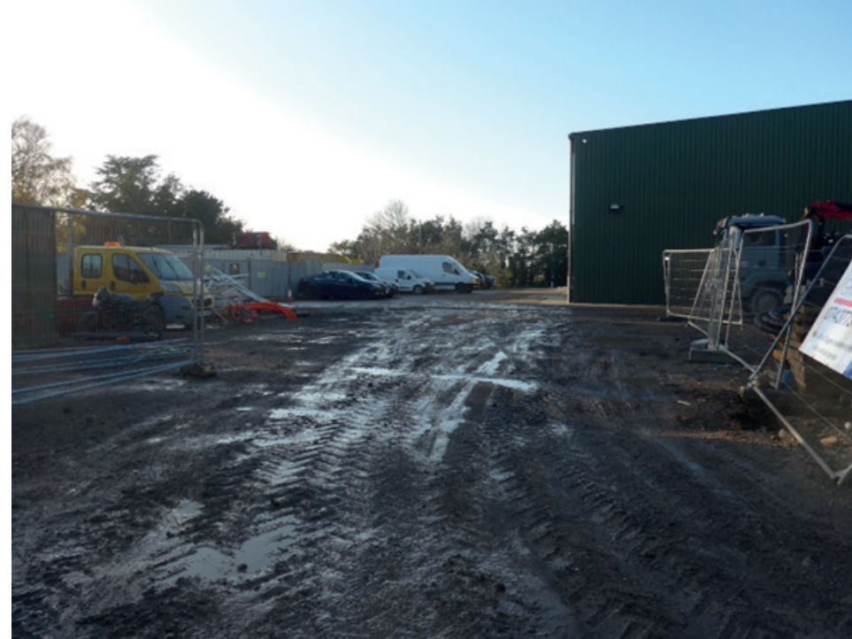
Site egress. Southwest corner of the site..
