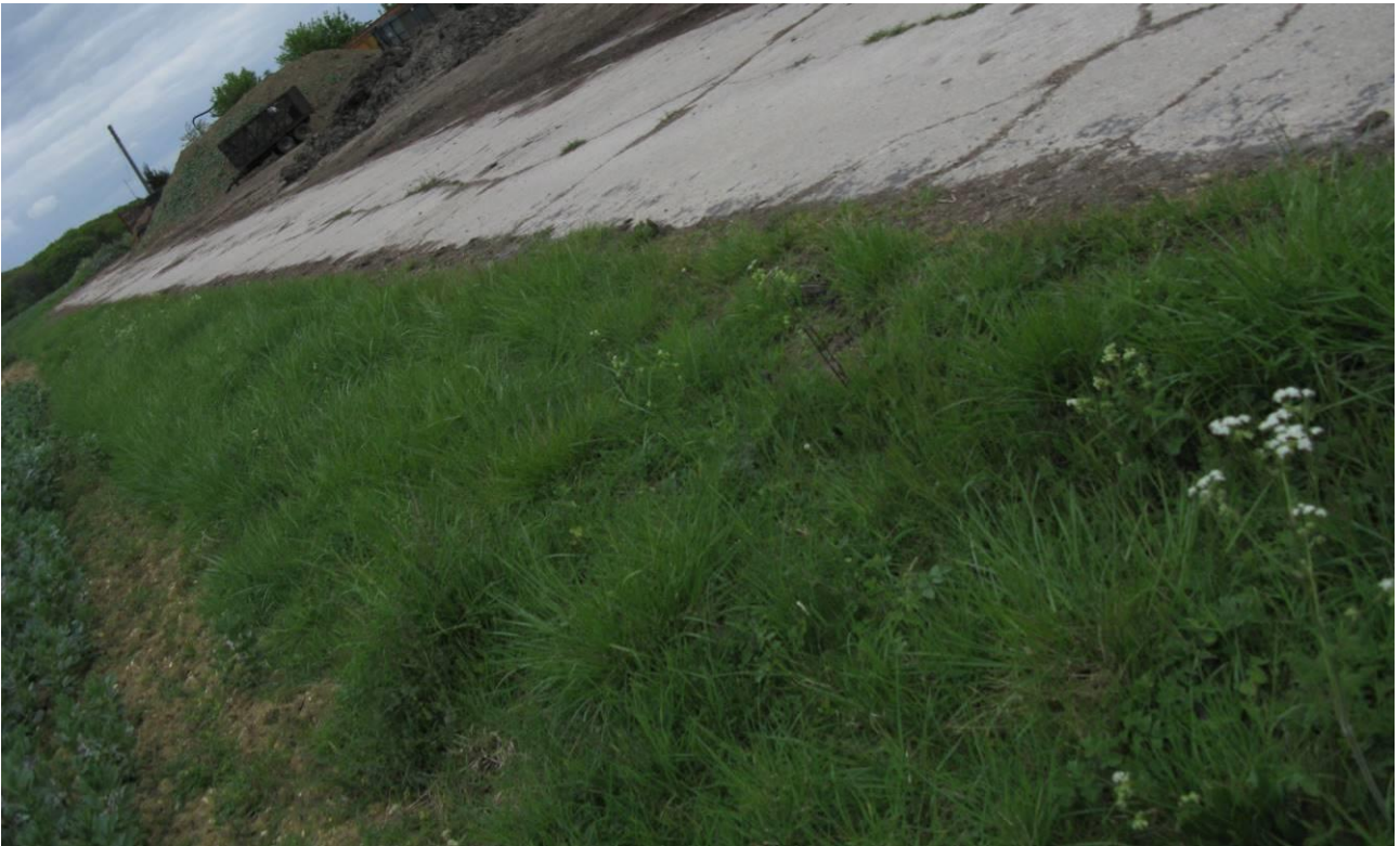
Narrow grassland strip with cow parsley and cranesbill near the northwest access road.
