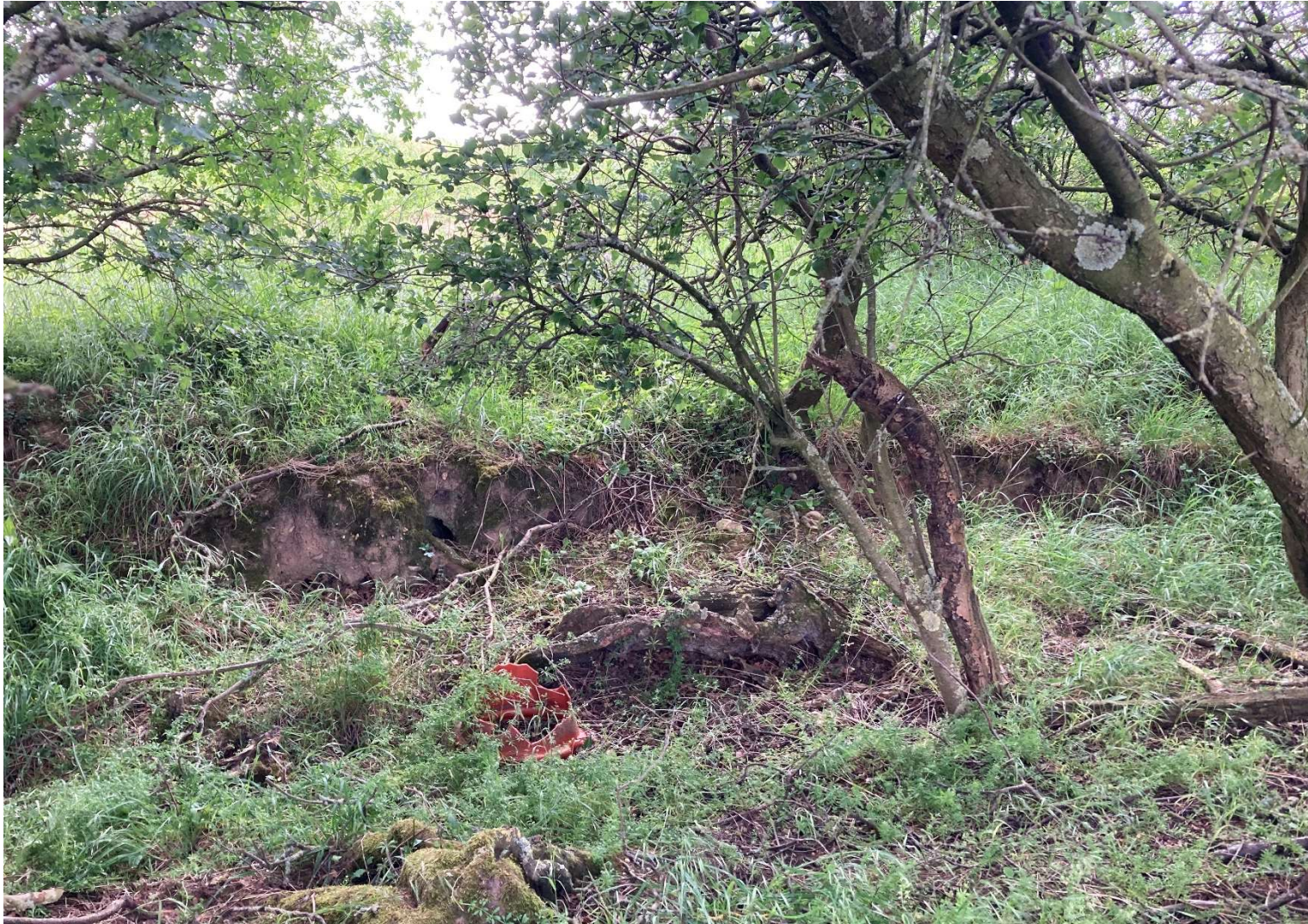
Photo 1 – instable ground approximately 3m behind the crest of the western quarry face (potential slope failure in the long term)
