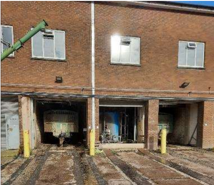
Photo 12: Digested sludge cake storage
