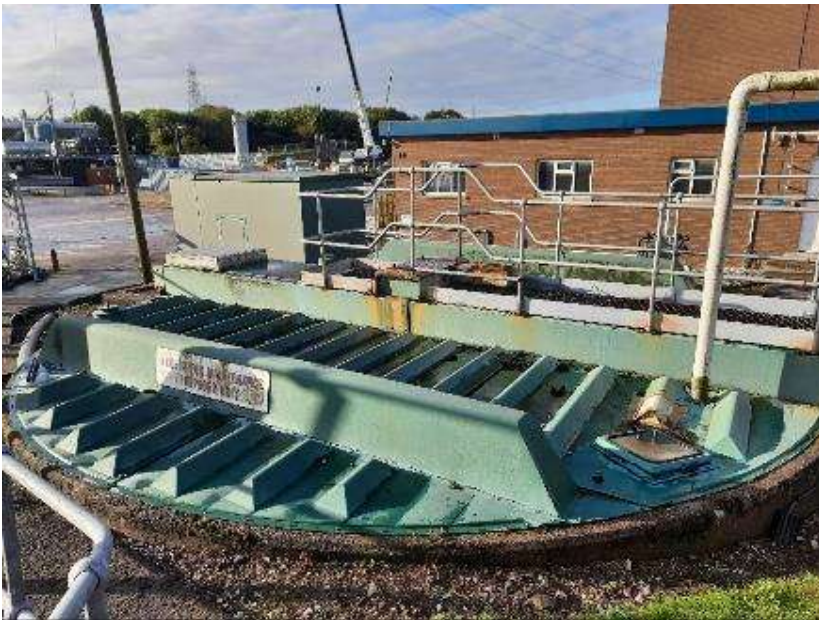
Photo 2: Raw sludge holding tank
