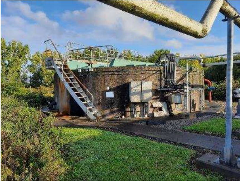
Photo 1: Raw sludge tank
