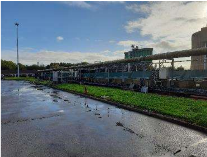
Photo 6: Thickened sludge tanks
