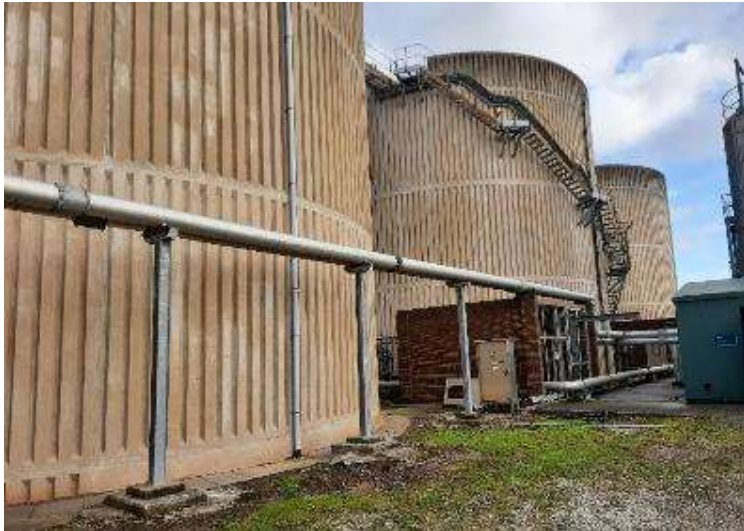
Photo 9: Mesophilic Anaerobic Digesters
