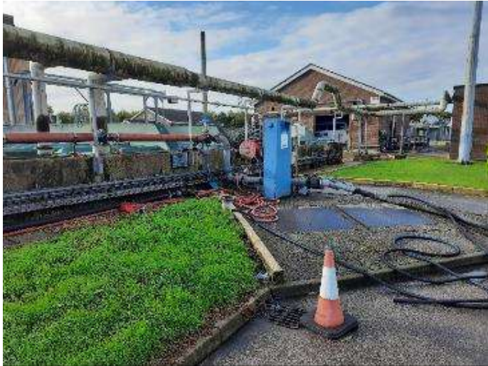
Photo 7: Thickened sludge import point
