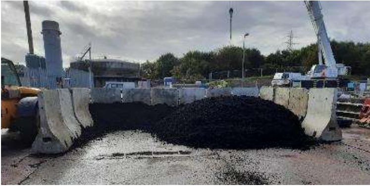
Photo 13: Contingency sludge cake storage pad
