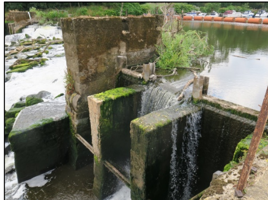
Photograph 20: Representative image of stonework [I]
