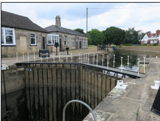
Photograph 5: Representative image of lock and buildings
