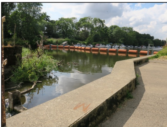
Photograph 7: Representative image of lock and buildings [A]
