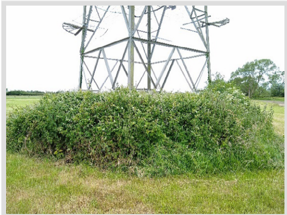
P – Stand of tall herbs at base of electricity pylon- photo June 2021
