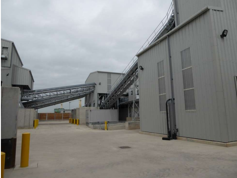
Photo 2: Enclosed waste treatment and covered conveyors
