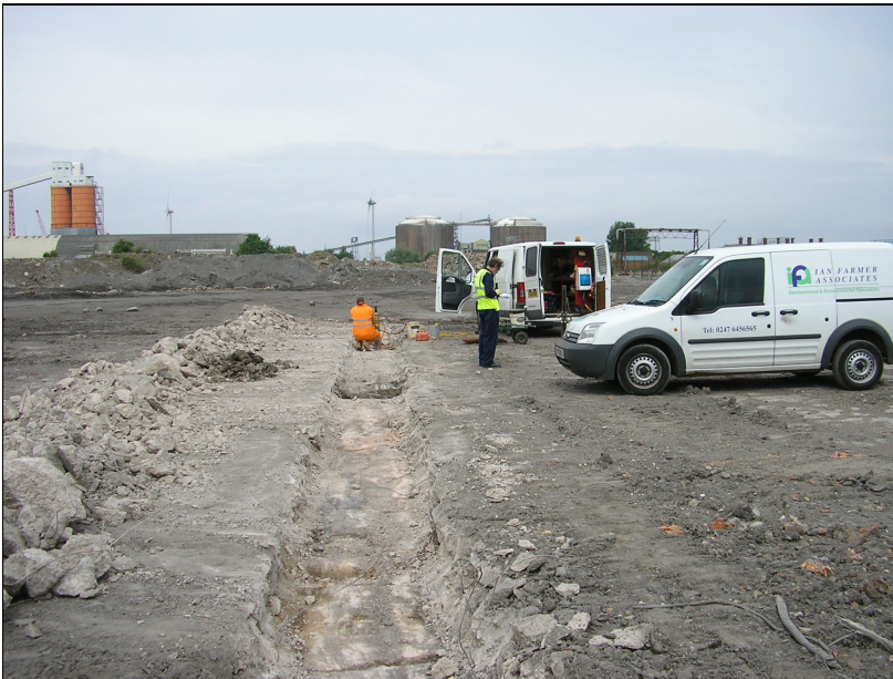
Plate 2 – Trench dug to expose potential asbestos containing concrete
