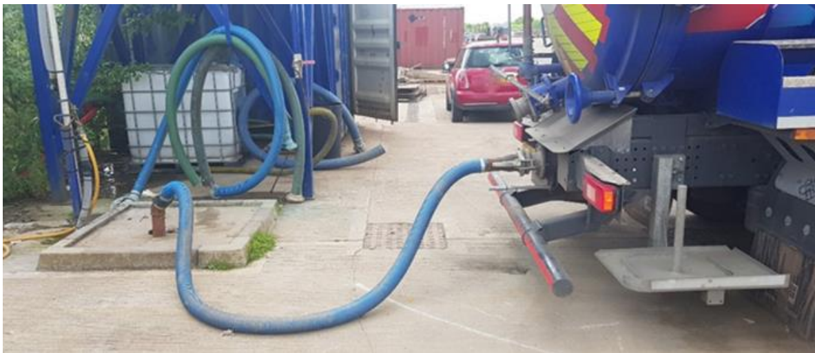
Example of discharge point
