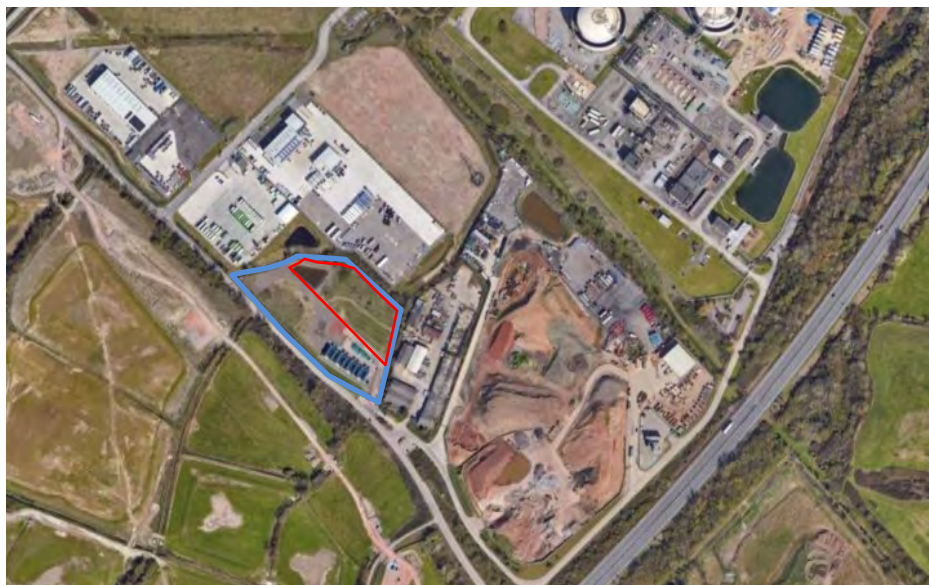
Figure 003: Existing Site Layout – Aerial Photograph
